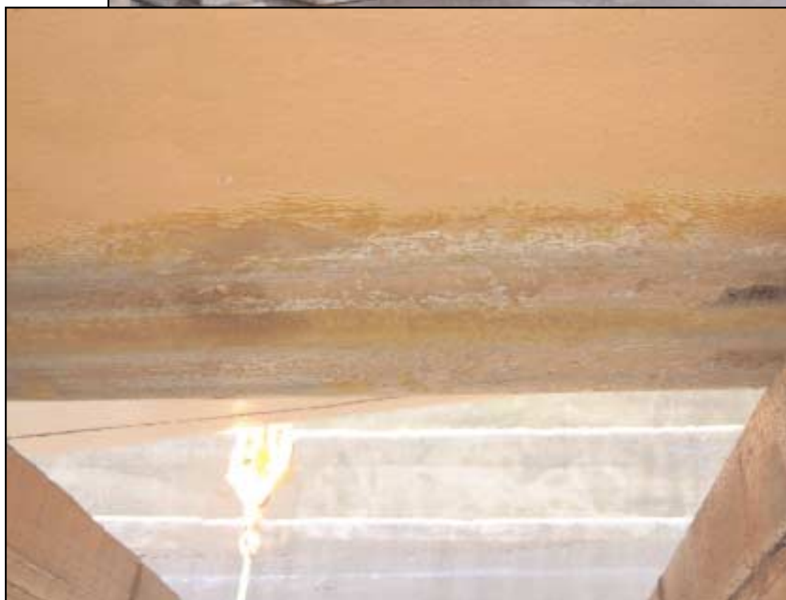
Small indentation damage to keel at aft end
