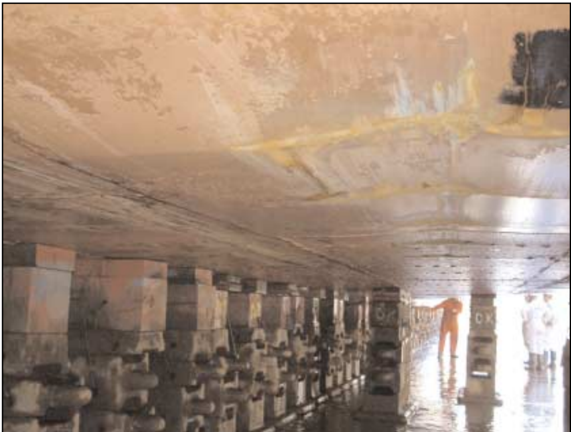
Indentation damage to Waverley's hull - port side midships, looking aft
