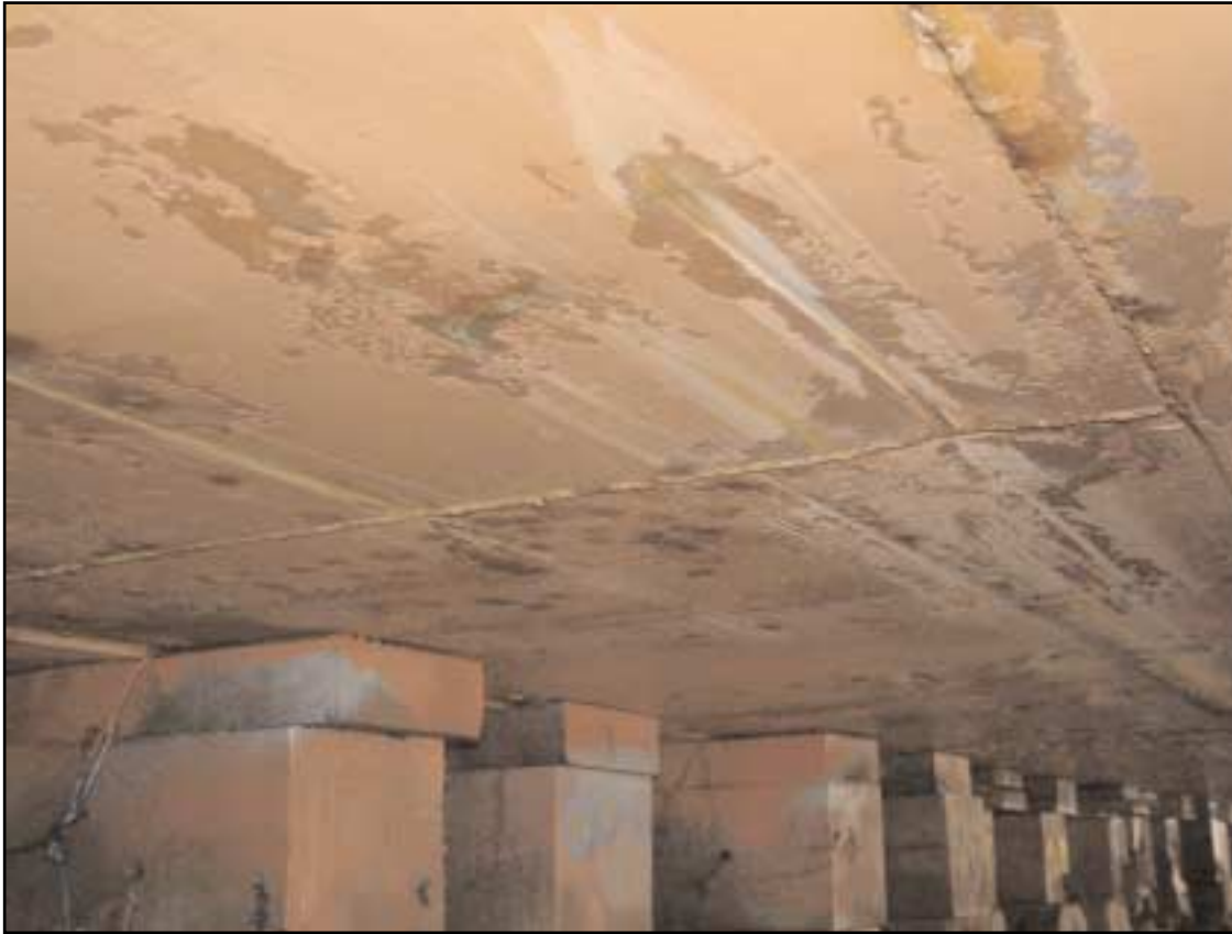
Scratching and scrape damage, port side, looking aft
