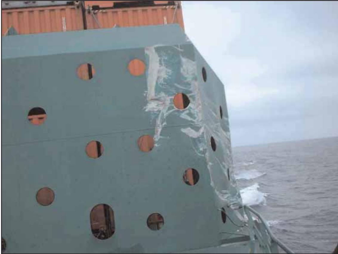
Damaged breakwater - Hyundai Dominion
