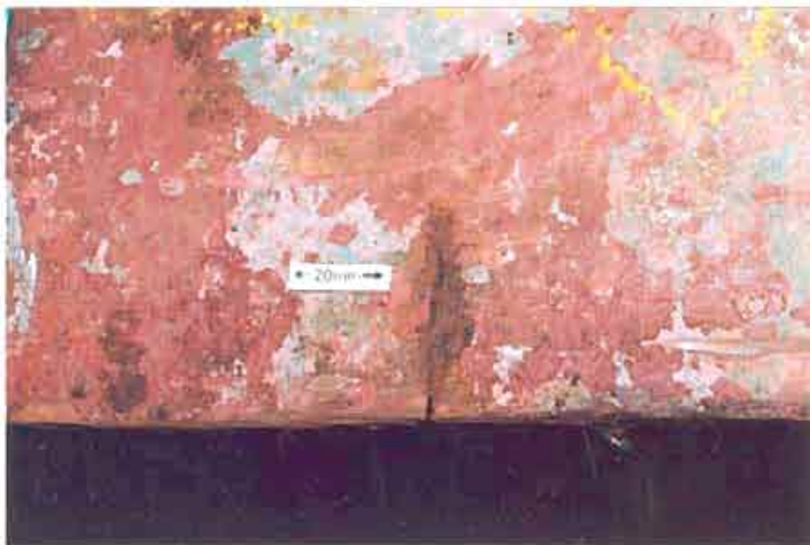
Figure 45: Detail of figure 44 showing second longitudinal crack.
