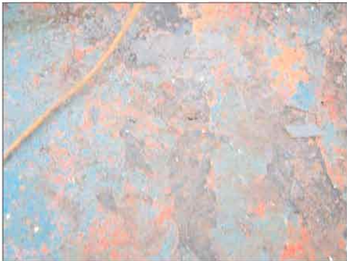
Area of flexing upper deck steelwork
