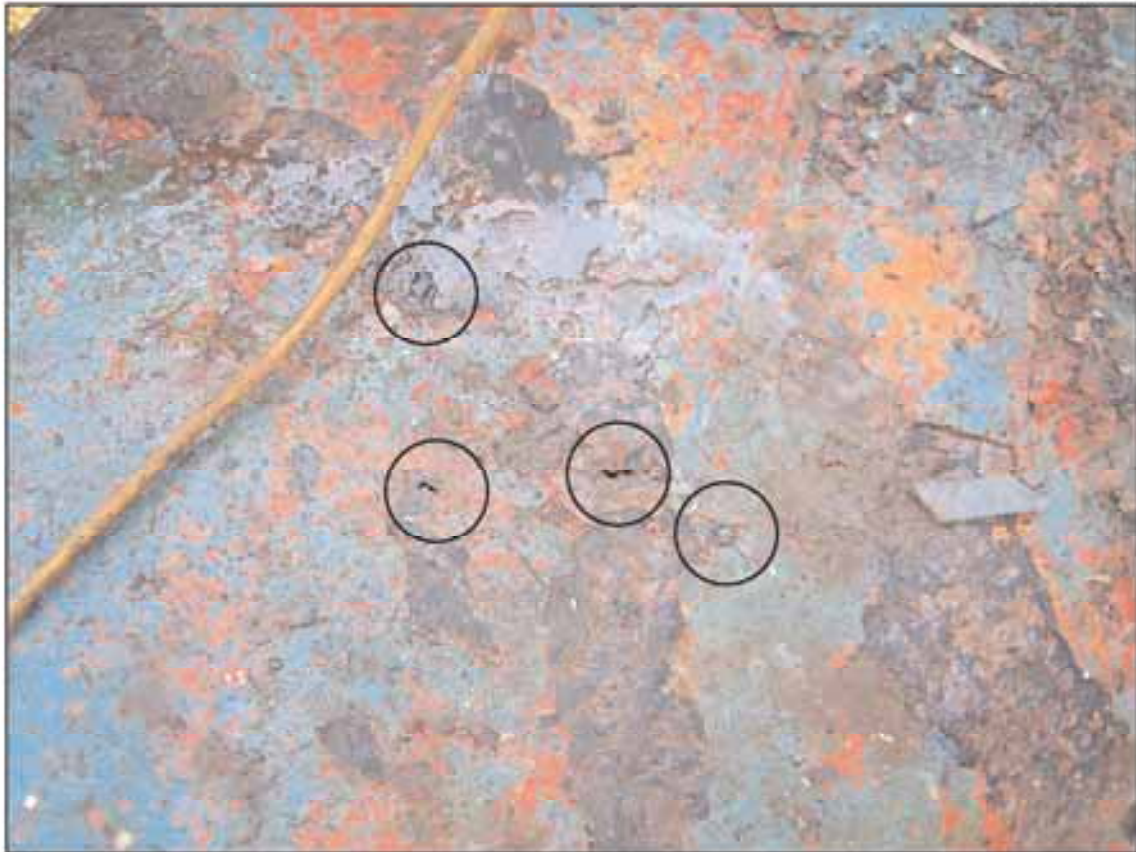
Perforations to upper deck above steering compartment
