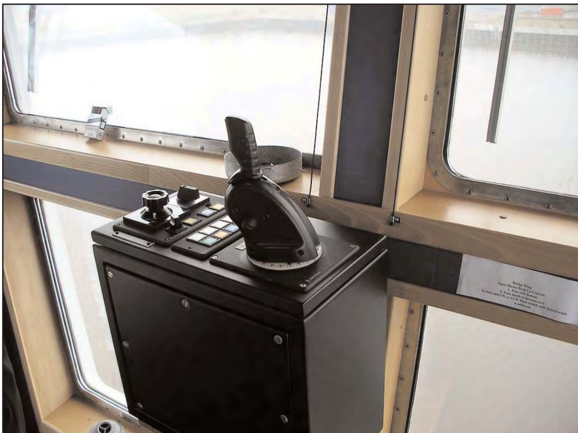
The second bridge wing thruster control handset
