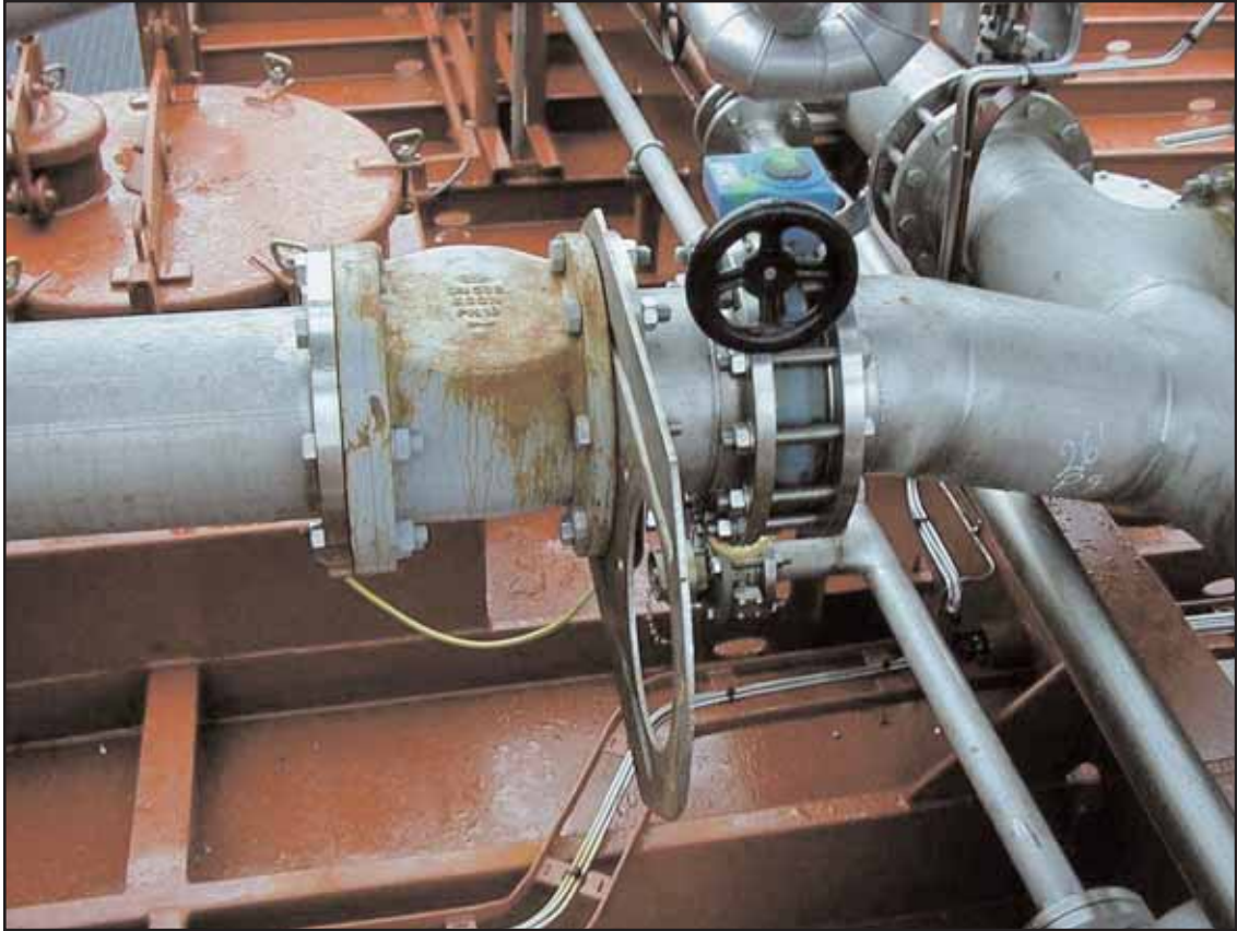
Spectacle plate in 'blanked' position
