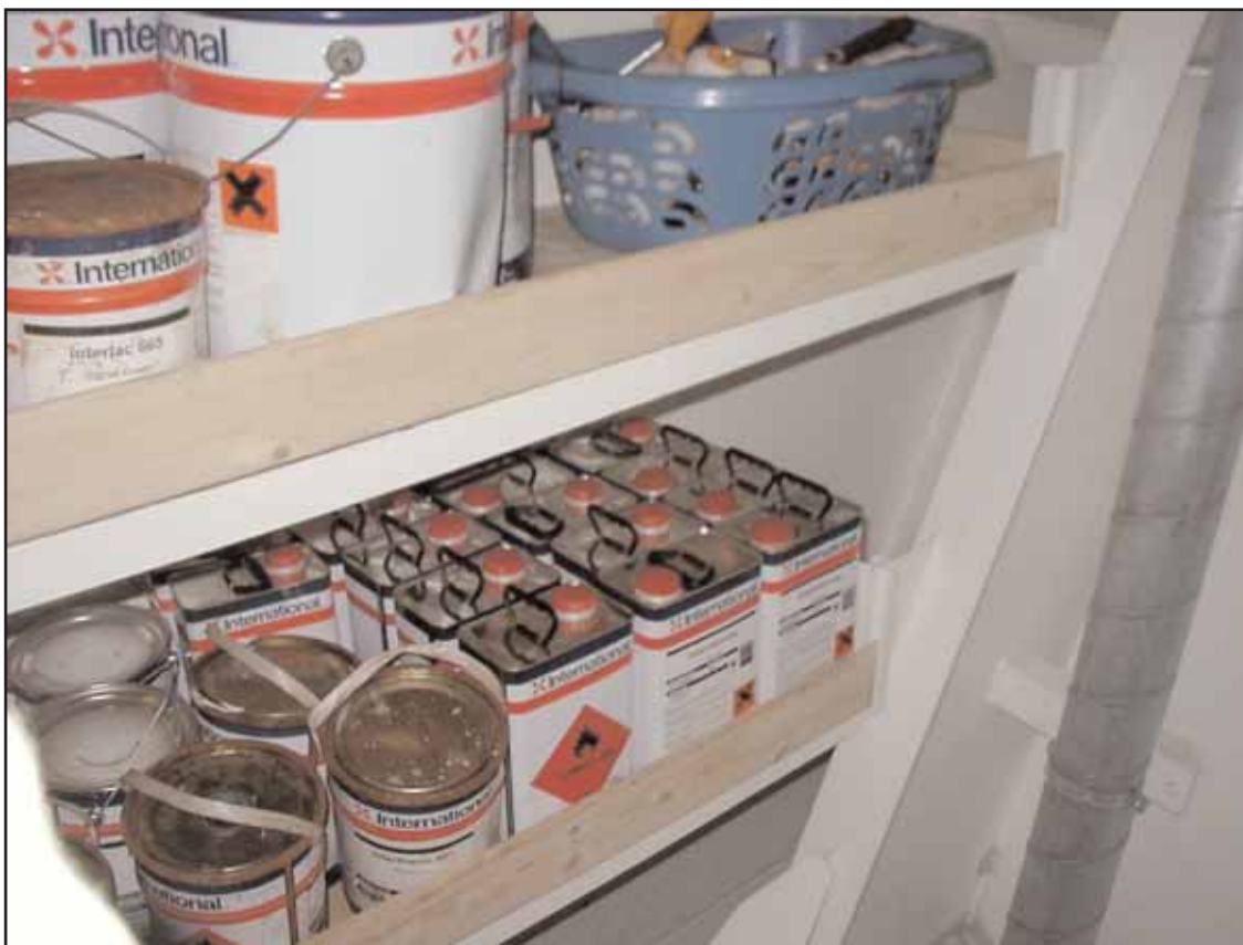
No damage internally to paint store
