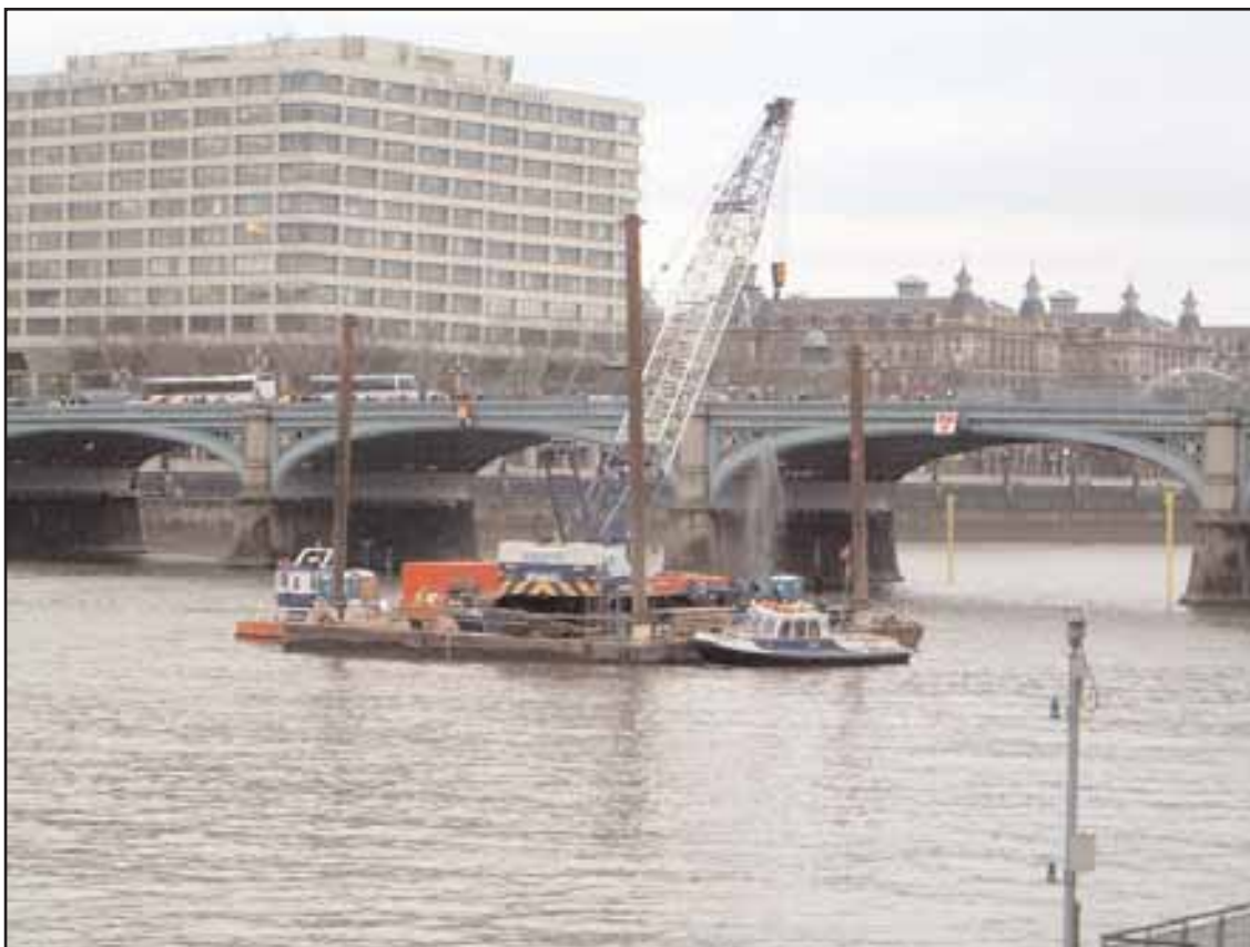
Construction work at Westminster Bridge
