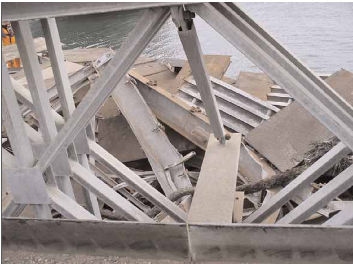
Linkspan damage
