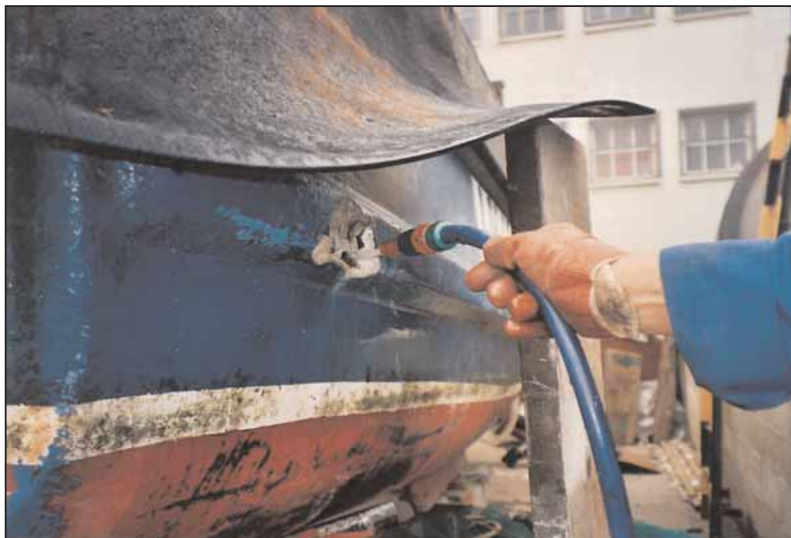
Hose test on damage
