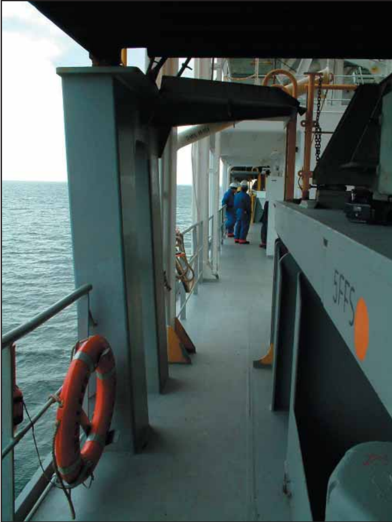
Pedestal support pre-accident
