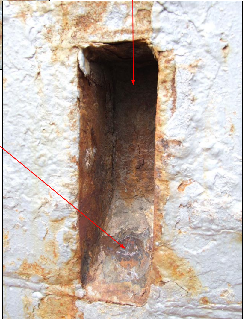
Securing pin pocket, starboard upper aft
