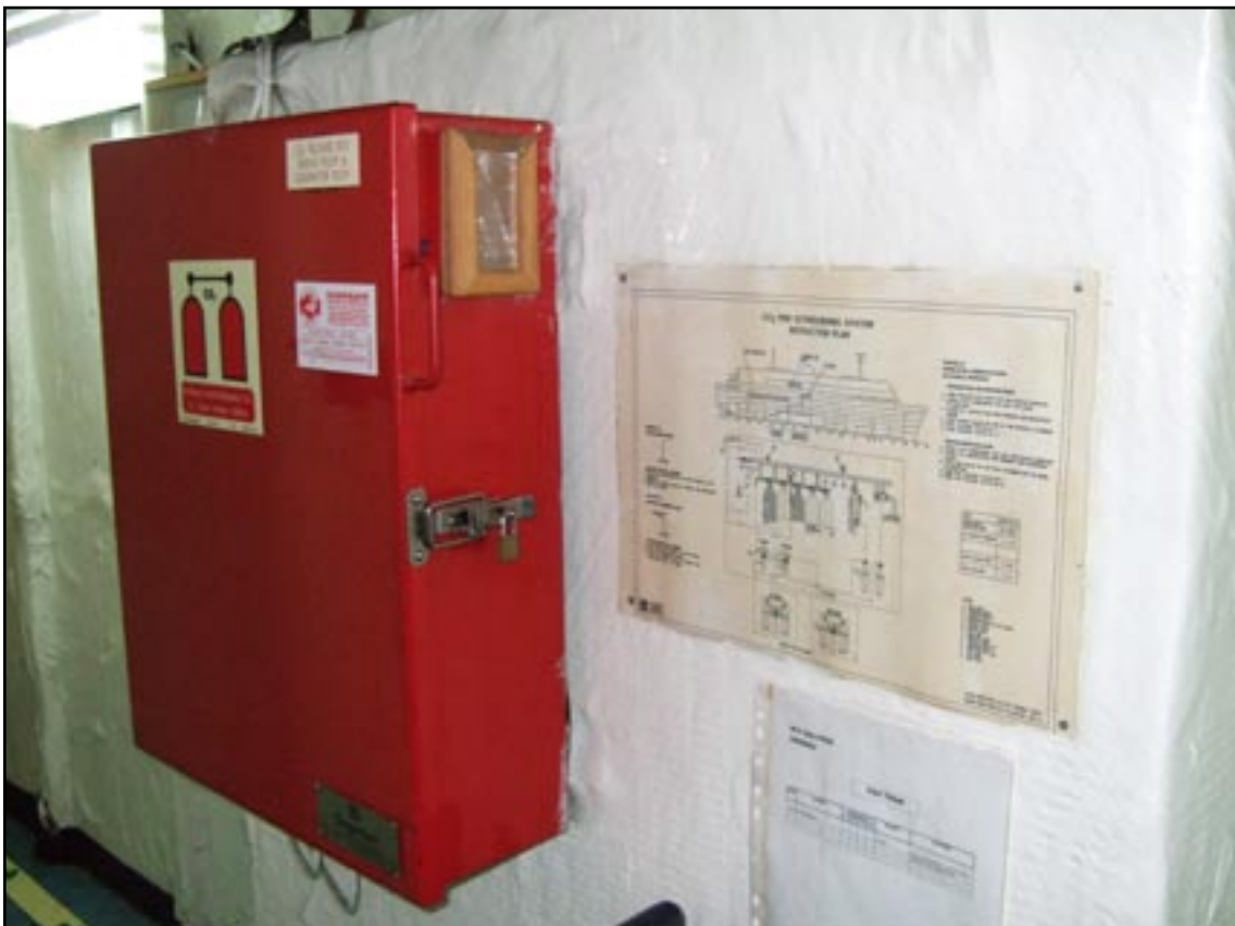
Remote CO2 release station for engine room
