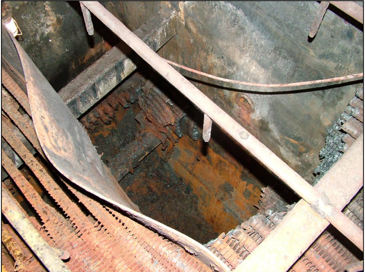
Location of damaged tubes, cut away to create exhaust gas path
