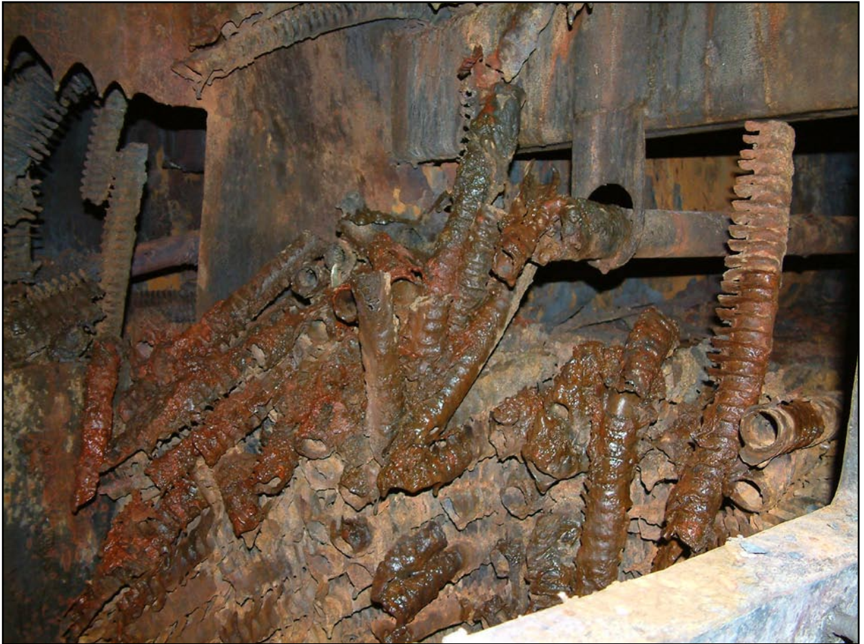
Damaged tubes in EGE
