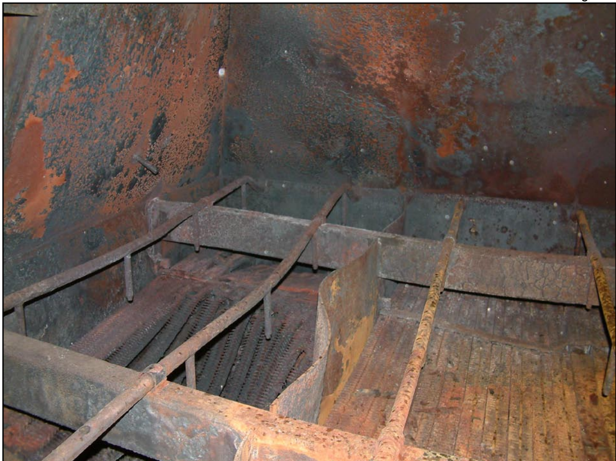
Water washing pipework and nozzles at the top of the EGE
