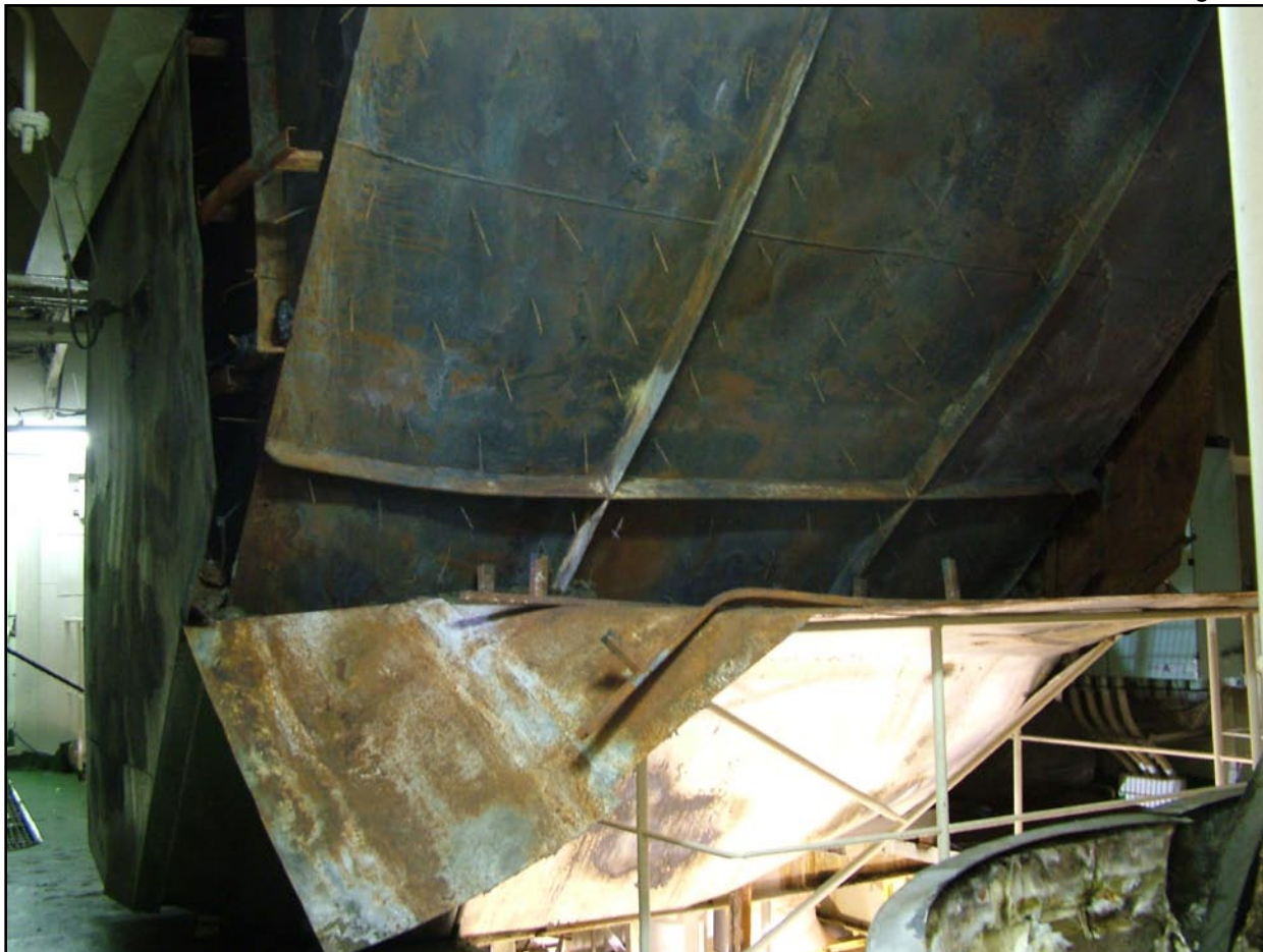
View of EGE and detached insulation
