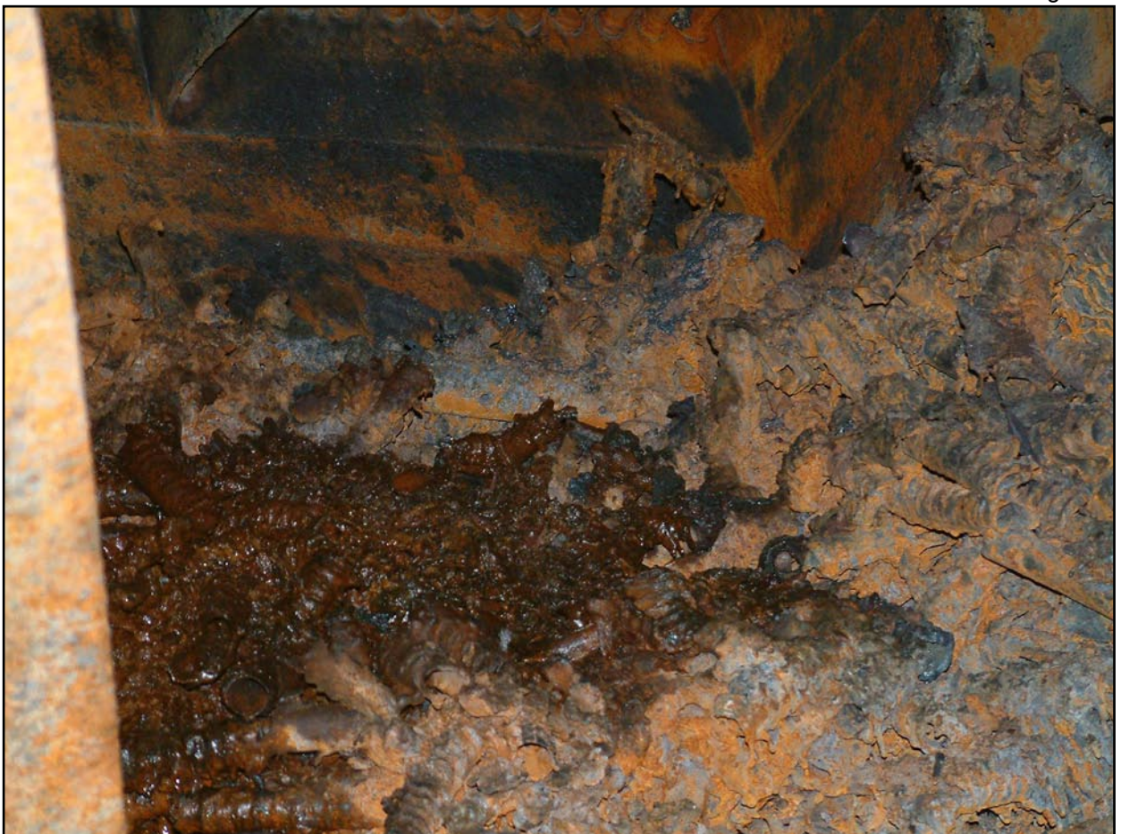
Debris at base of EGE trunking
