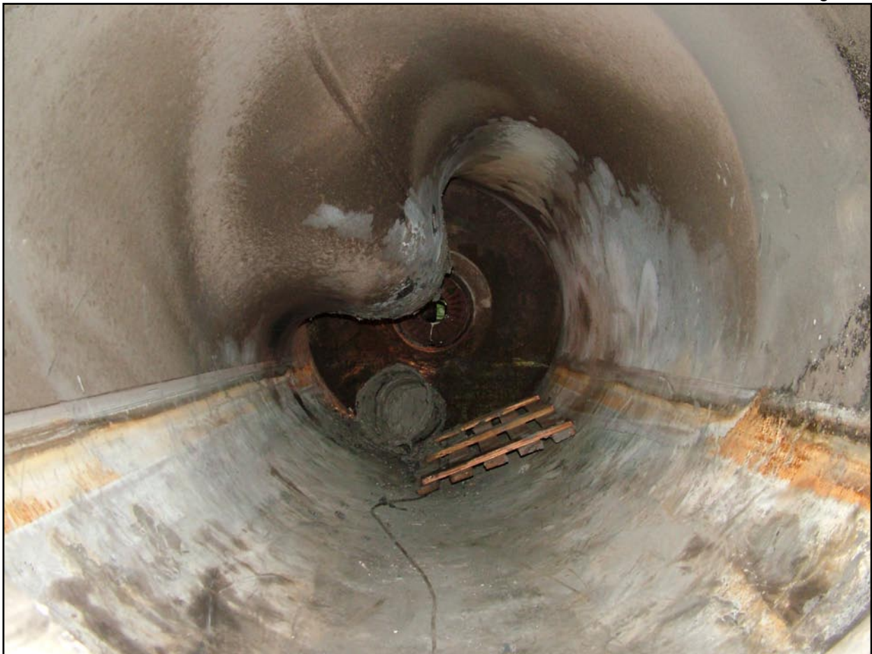
Auxiliary boiler - distorted furnace tube
