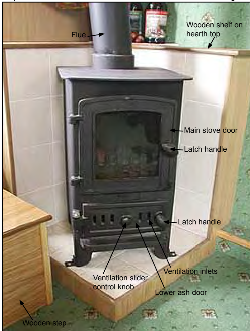
Stove installation on board another Triton narrowboat
