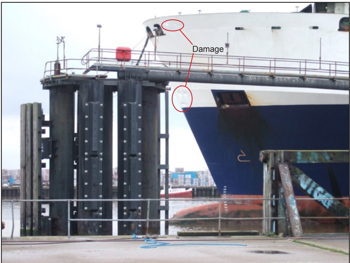
Damage to Ursine (top) and Pride of Bruges (bottom)
