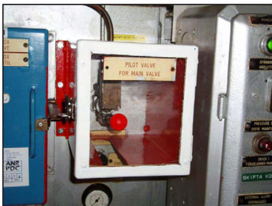
Protective enclosure to main release valve on CO 2 room control panel
