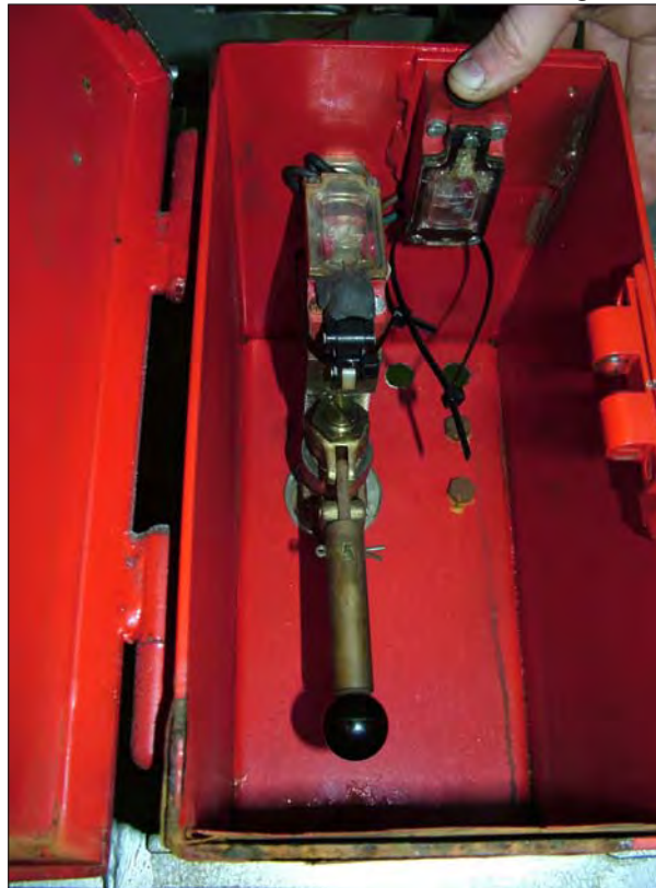
Distribution valve pilot release control lever
