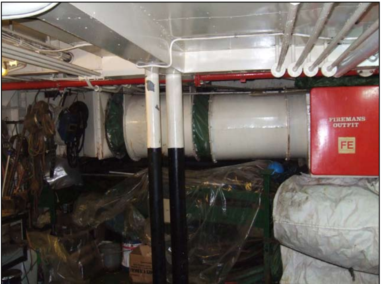
Forward store - port cargo ventilation trunking
