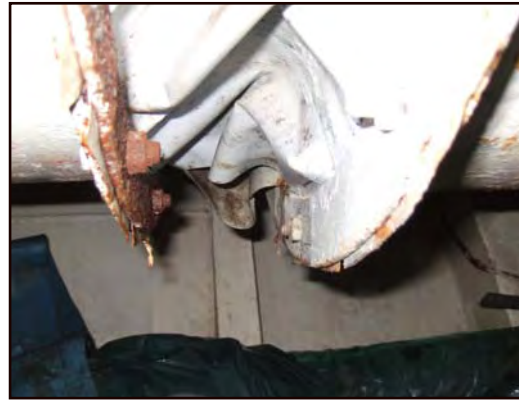
Cut ventilation duct
