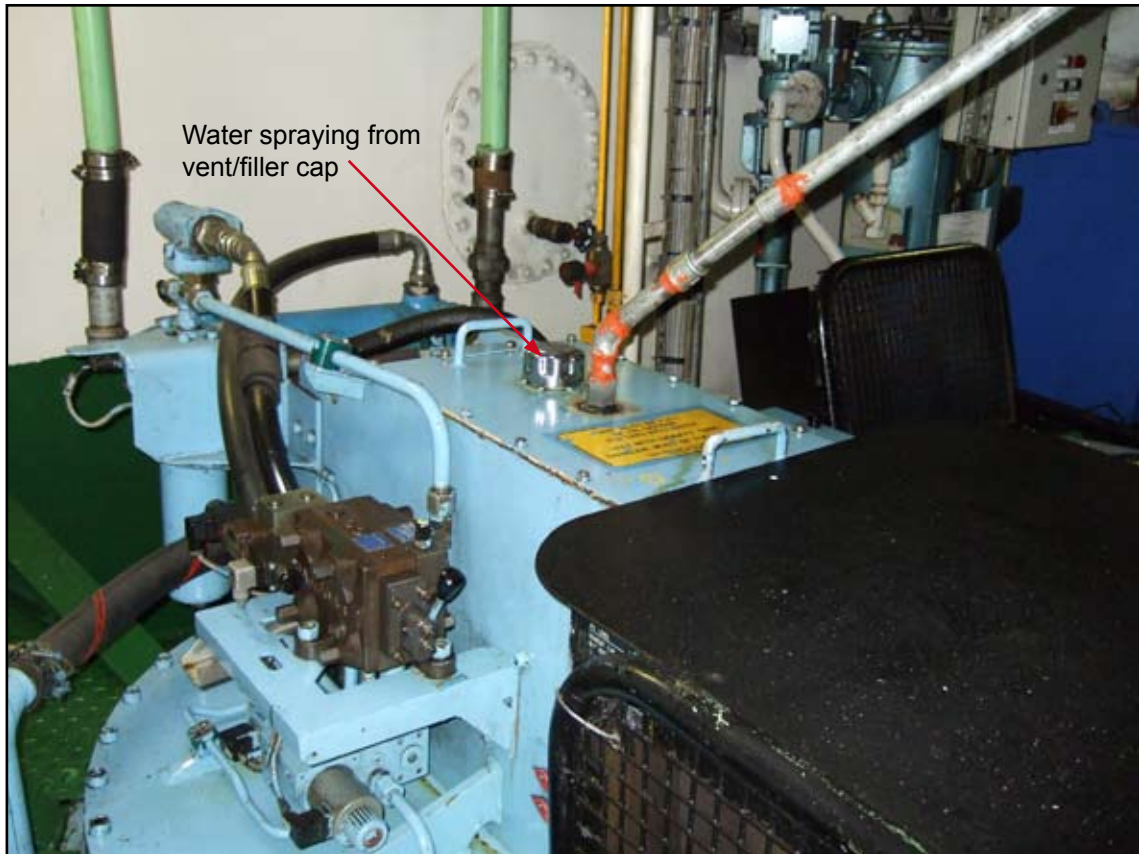
Photograph showing position of water ingress
