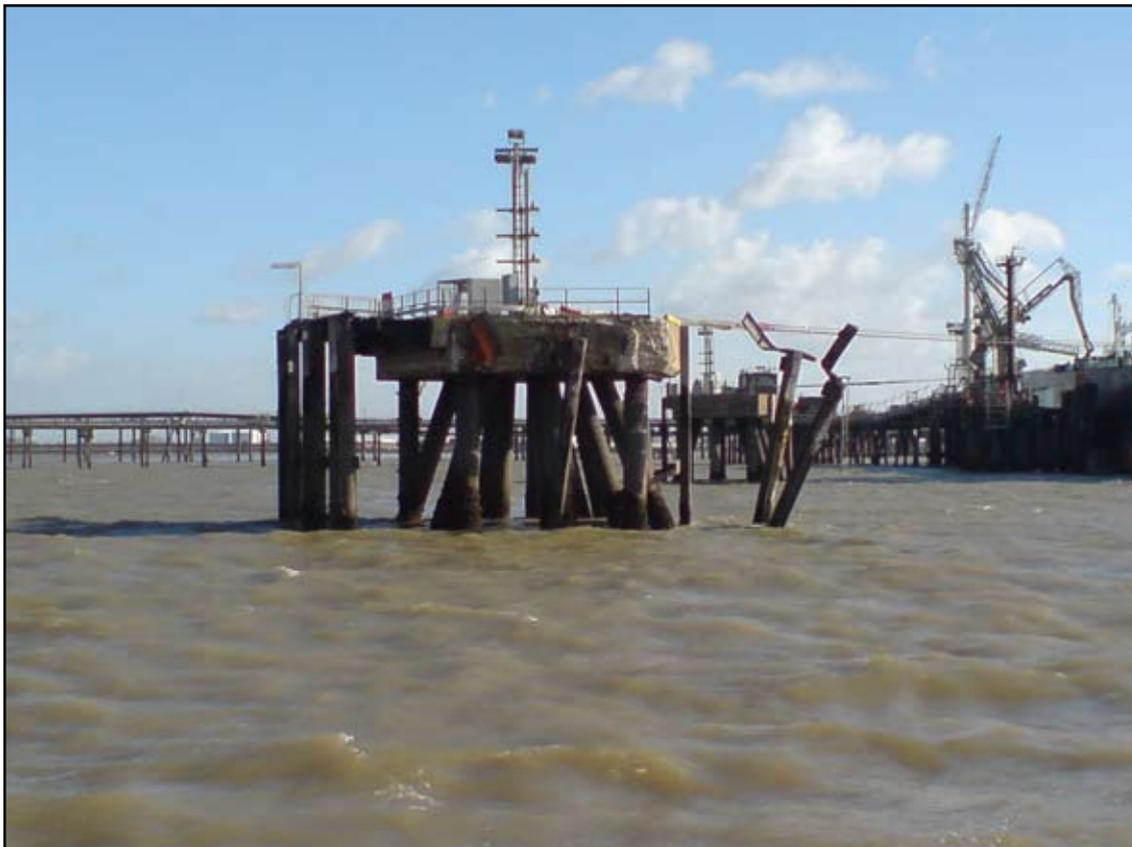
Damage to MD 41 mooring structure and stern lines leading to *Thornbury*
