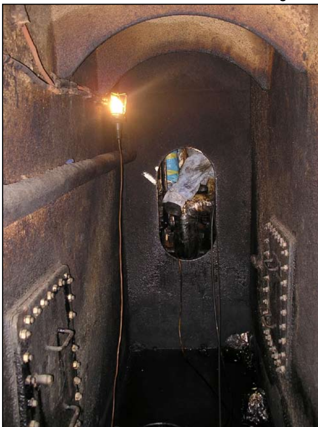
Entrance to the cofferdam (view from cofferdam)
