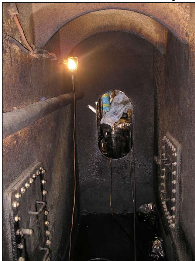
Entrance to the cofferdam (view from cofferdam)
