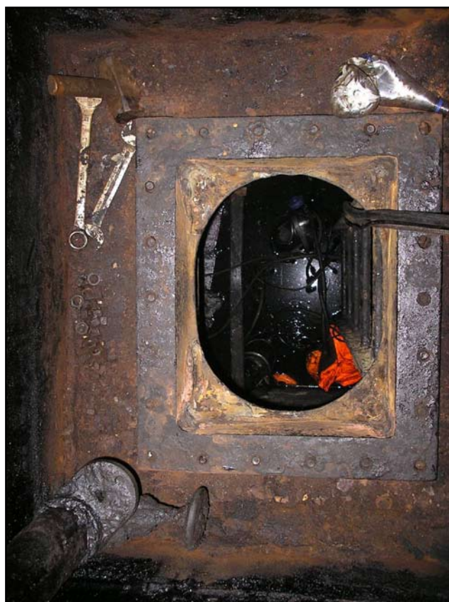
No.4 port outer double bottom tank manhole
