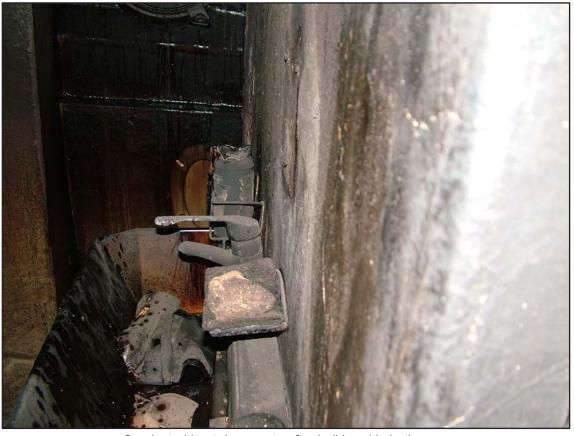
Conducted heat damage to after bulkhead in bathroom
