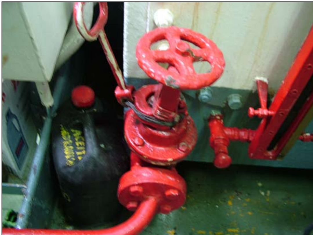
Quick shut-off valve lashed in the "open" position
