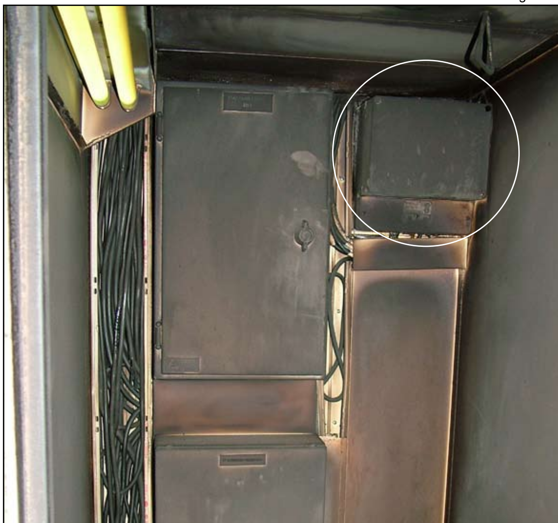
Location of fire detection system control box
