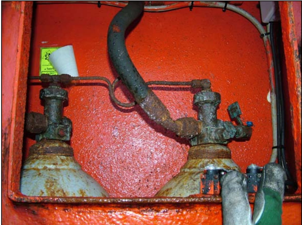
Corroded CO 2 bottle pipework
