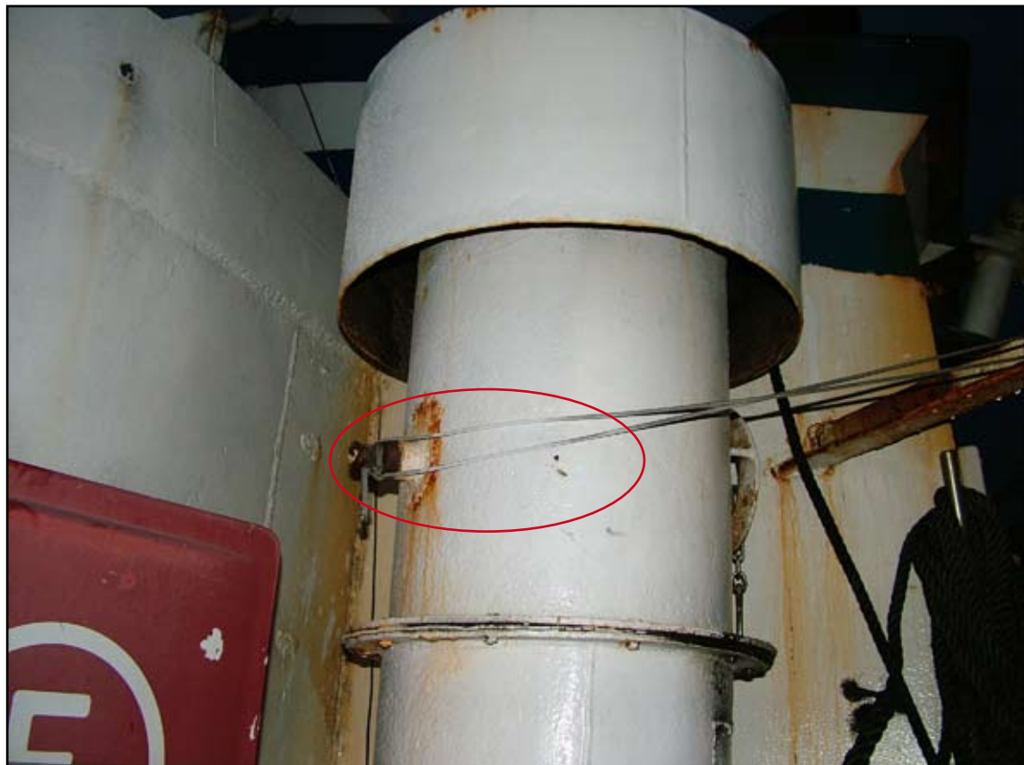
Ventilation shut-off flap valve obstructed by lashings
