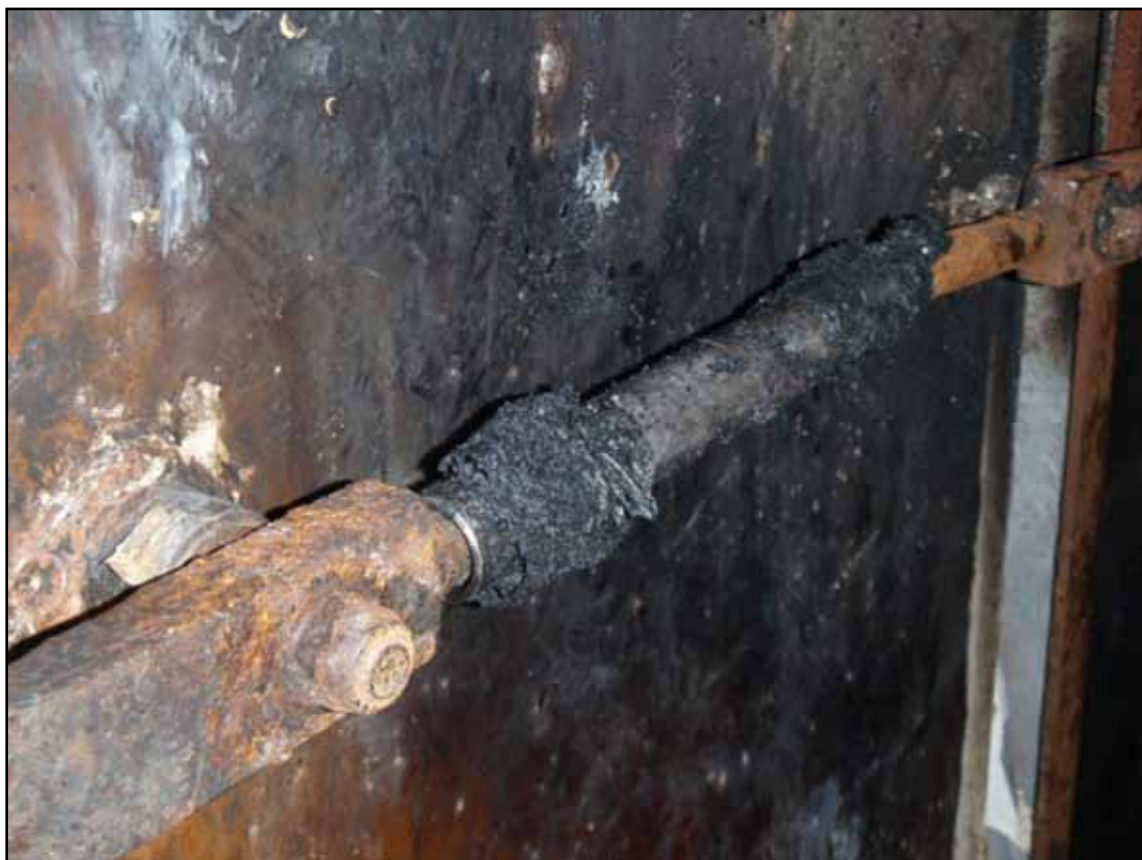
Example of the scaffolding tube used to secure two internal dogs
