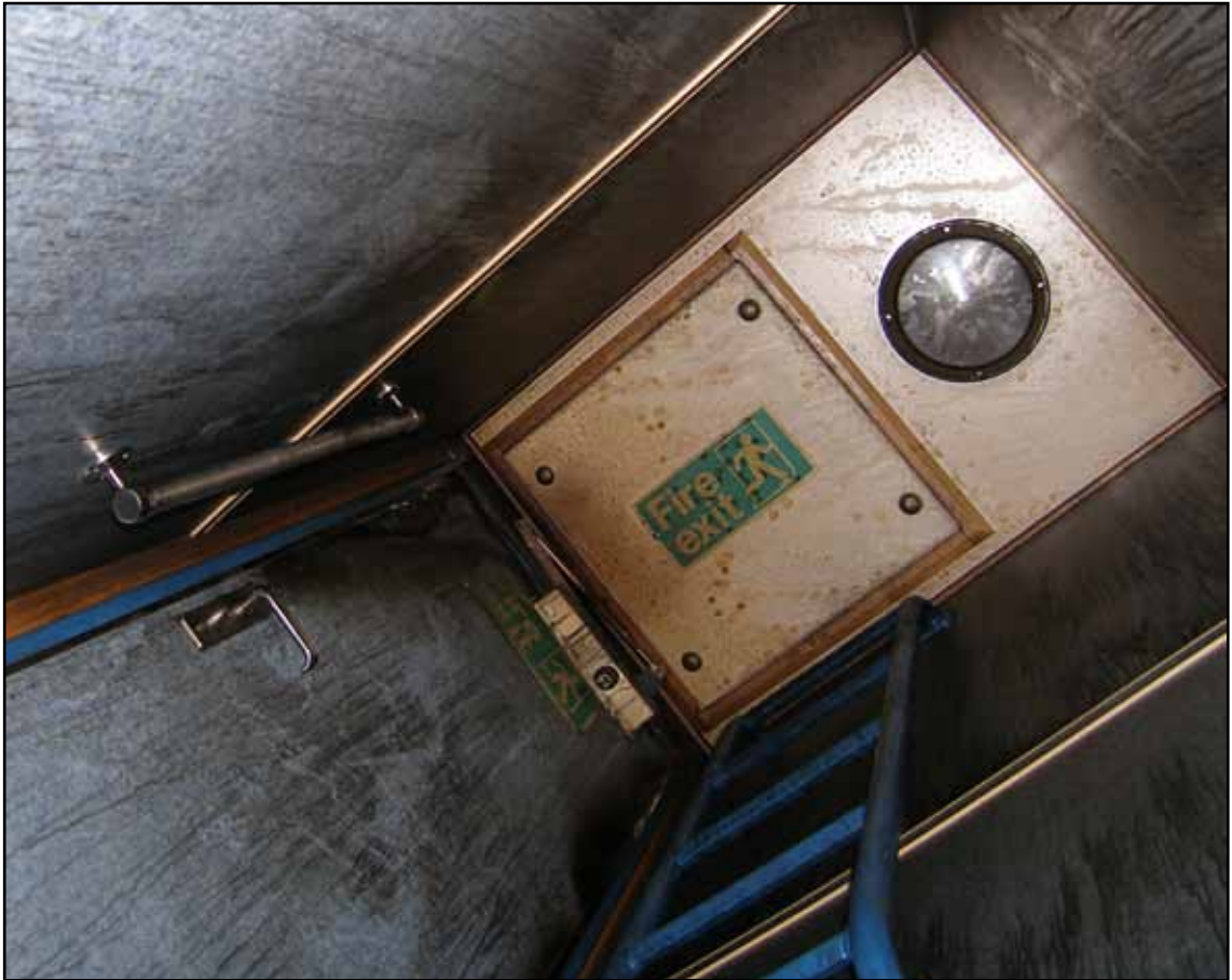
Internal deck head panel covering the escape hatch
