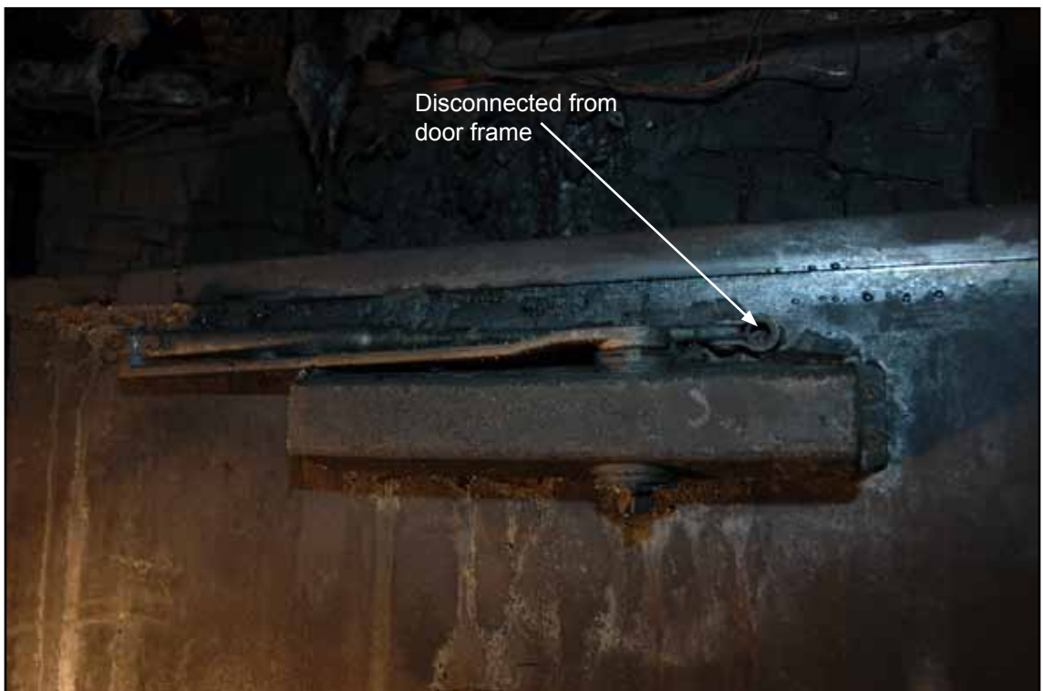
Galley fire door self-closing mechanism
