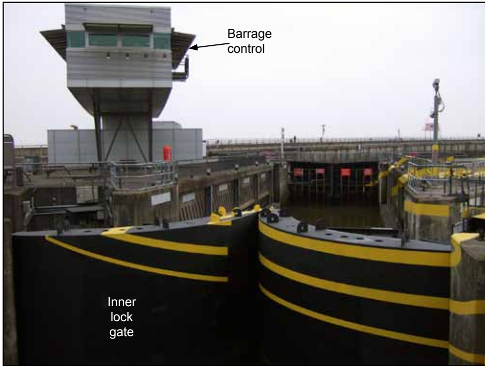
Cardiff Bay barrage locks
