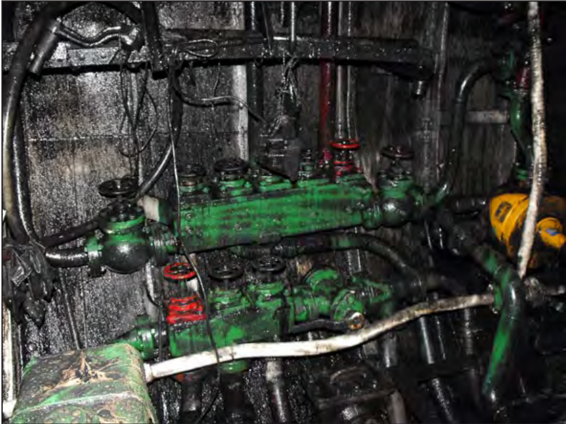
Fire main valves on the aft suction and discharge valve chests
