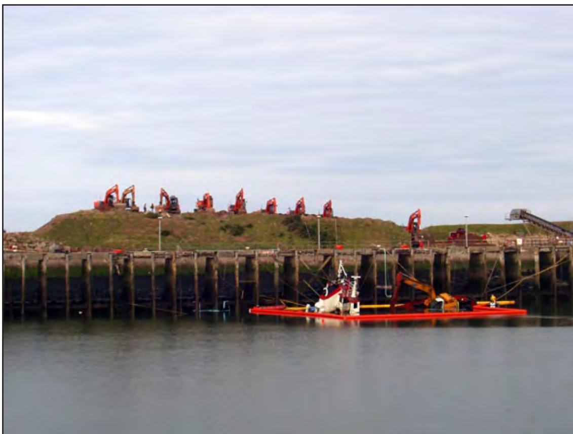
Excavators used to stabilise Abigail H
