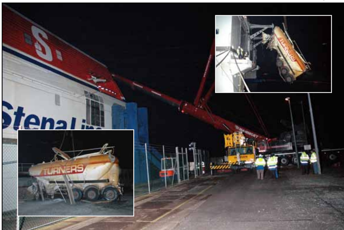
Road tanker recovery
