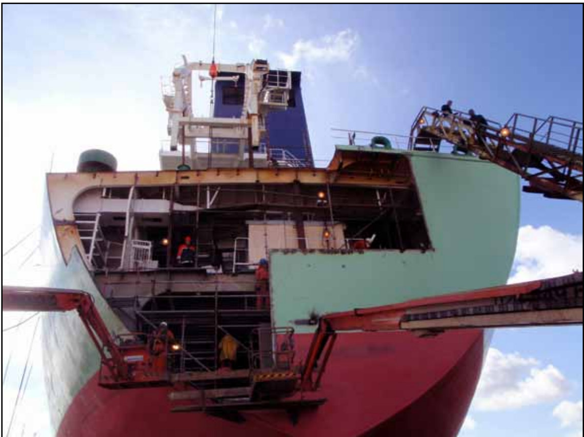
Repair work to BW Orinoco
