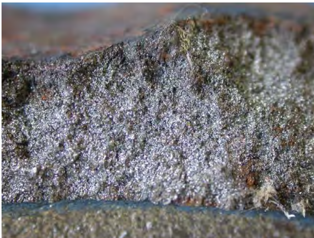
Figure 59: Detail of figure 58, showing fracture surface features consistent with a cast iron.
