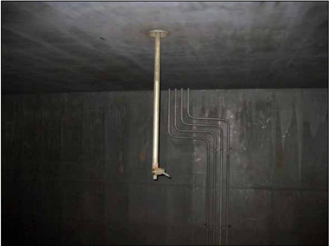
Gunclean 7000S fixed tank washing machine
