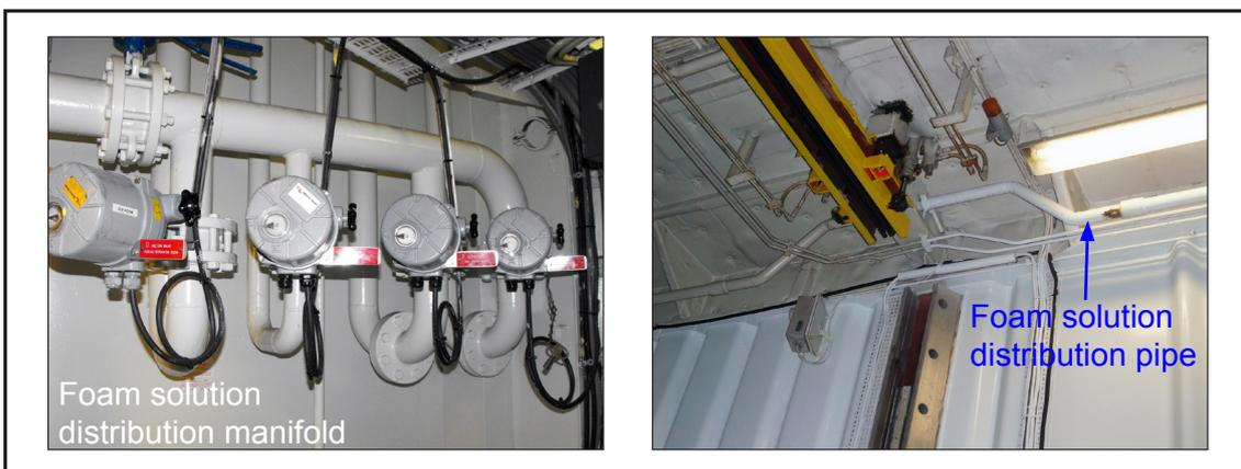
The debris found in the nozzles and piping is most likely to have been rust and scale that had built up in sections of pipe in which water and/or foam solution had previously been trapped. This debris would then have been distributed along the pipes and into the nozzles during the annual blow through tests and when the system was operated. The resulting blockages were sufficient to prevent the aspiration of the foam solution.
