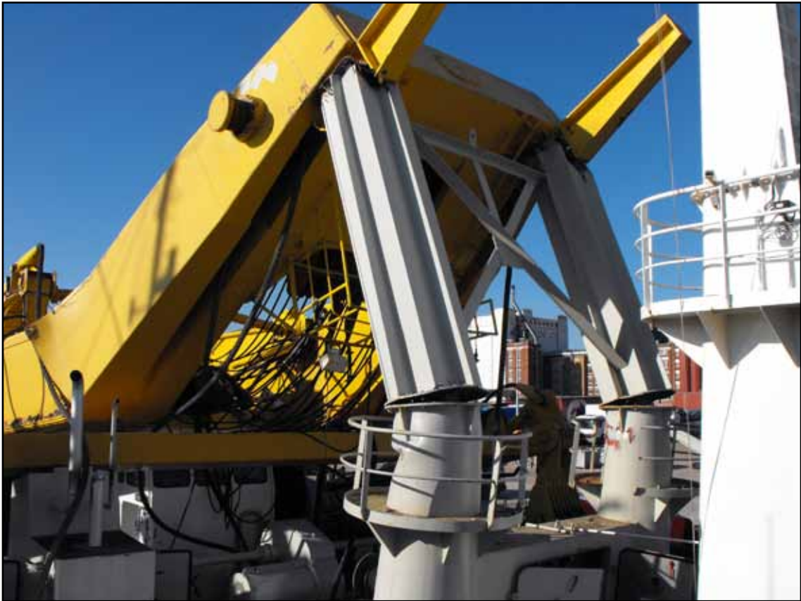
Buckling to the 'A' frame and its foundation
