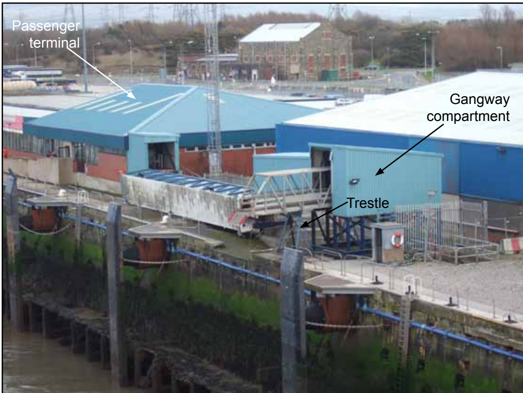
Passenger terminal and access structure
