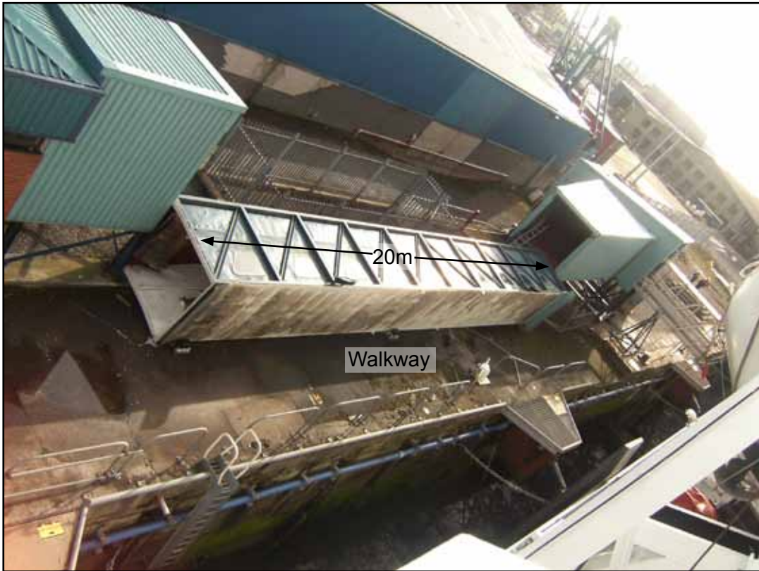
Passenger access structure
