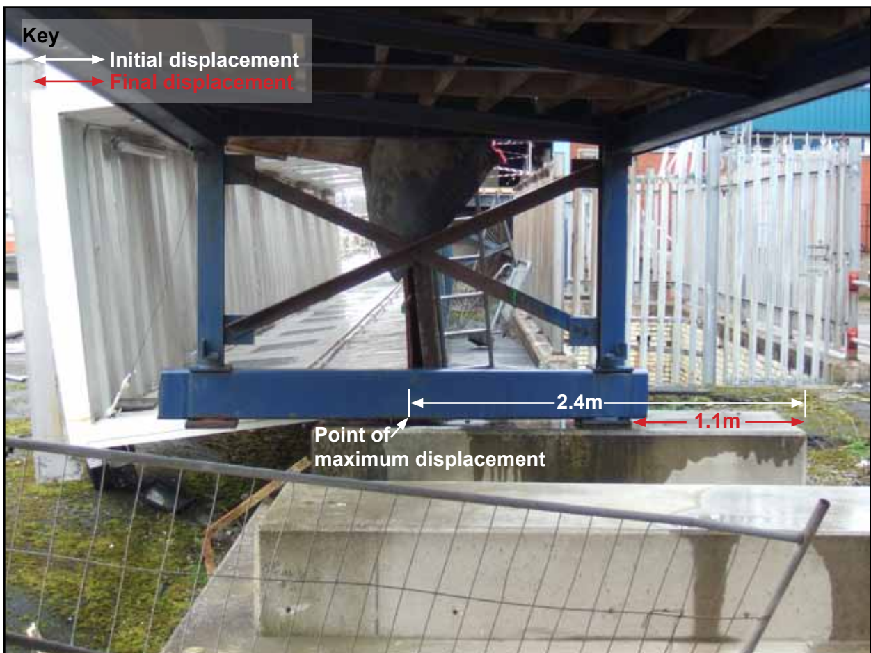
Movement of gangway compartment showing support frame in its final position after the accident
