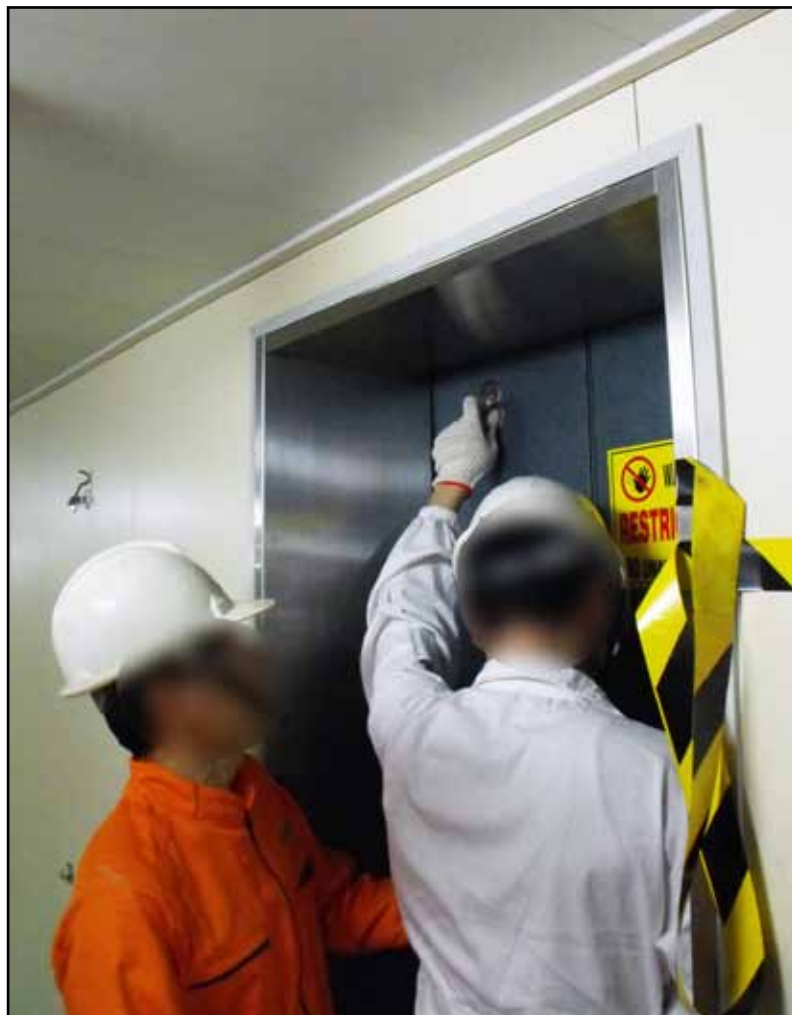
Lift shaft door manual opening
