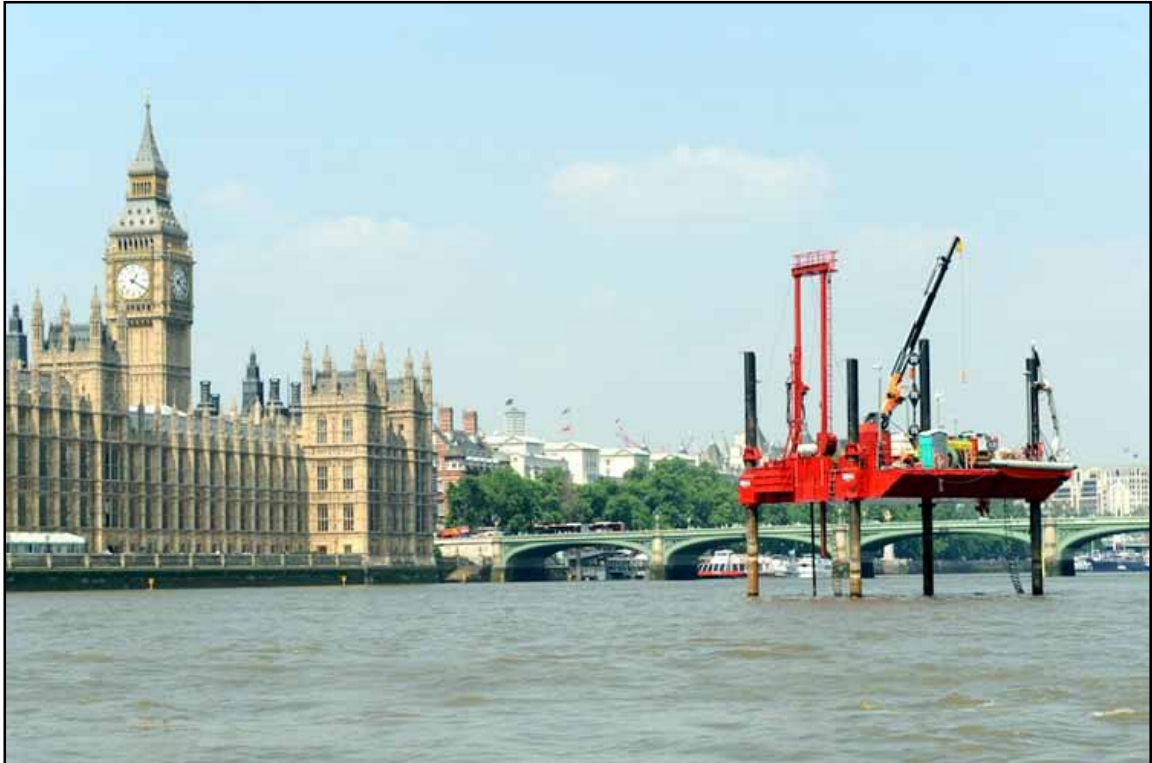
Fugro Seacore jack-up rig operating on River Thames
