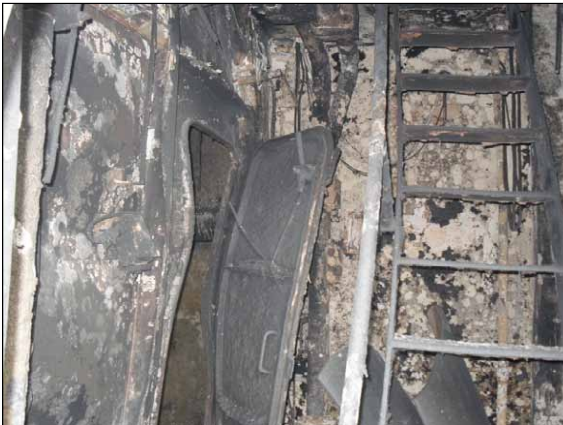
Example of distortion in the SUS tower
