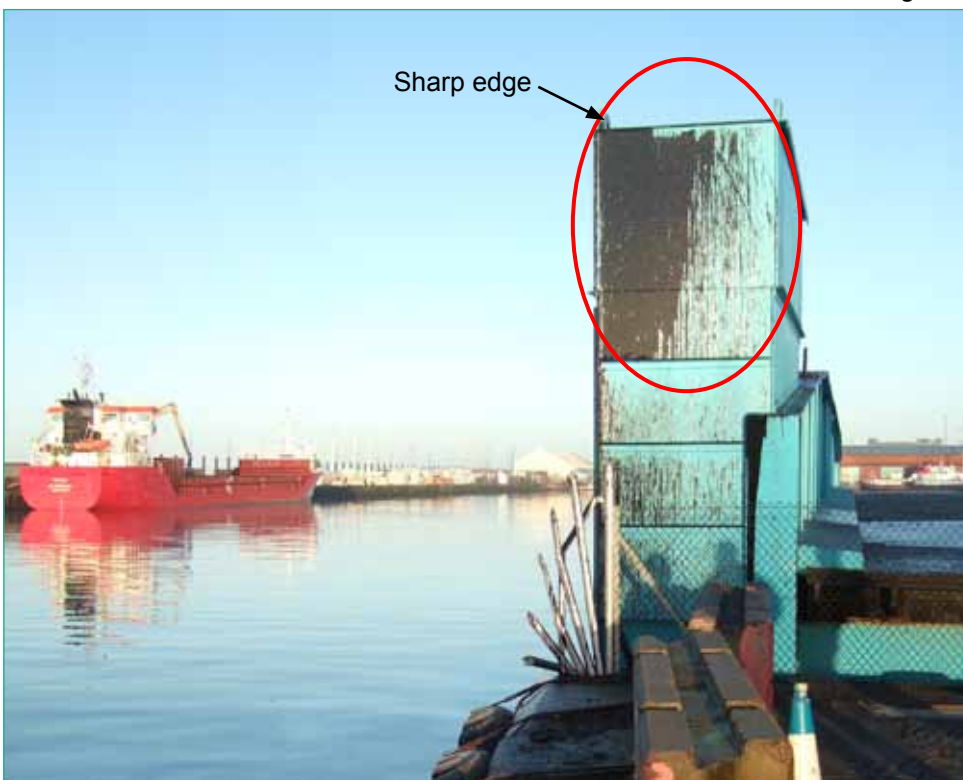
Swing bridge showing counterweight
