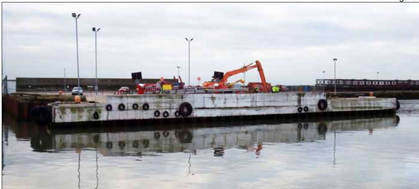
Western wall of passageway
