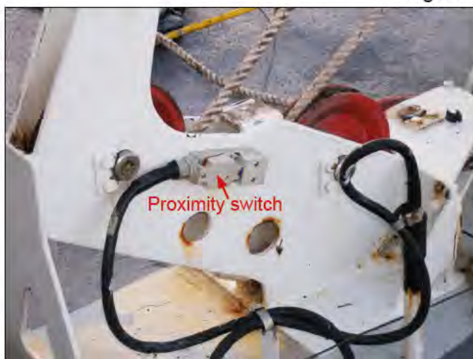
Proximity switch on davit
