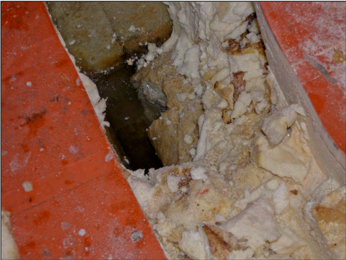
Figure 10: Free water in buoyancy space
