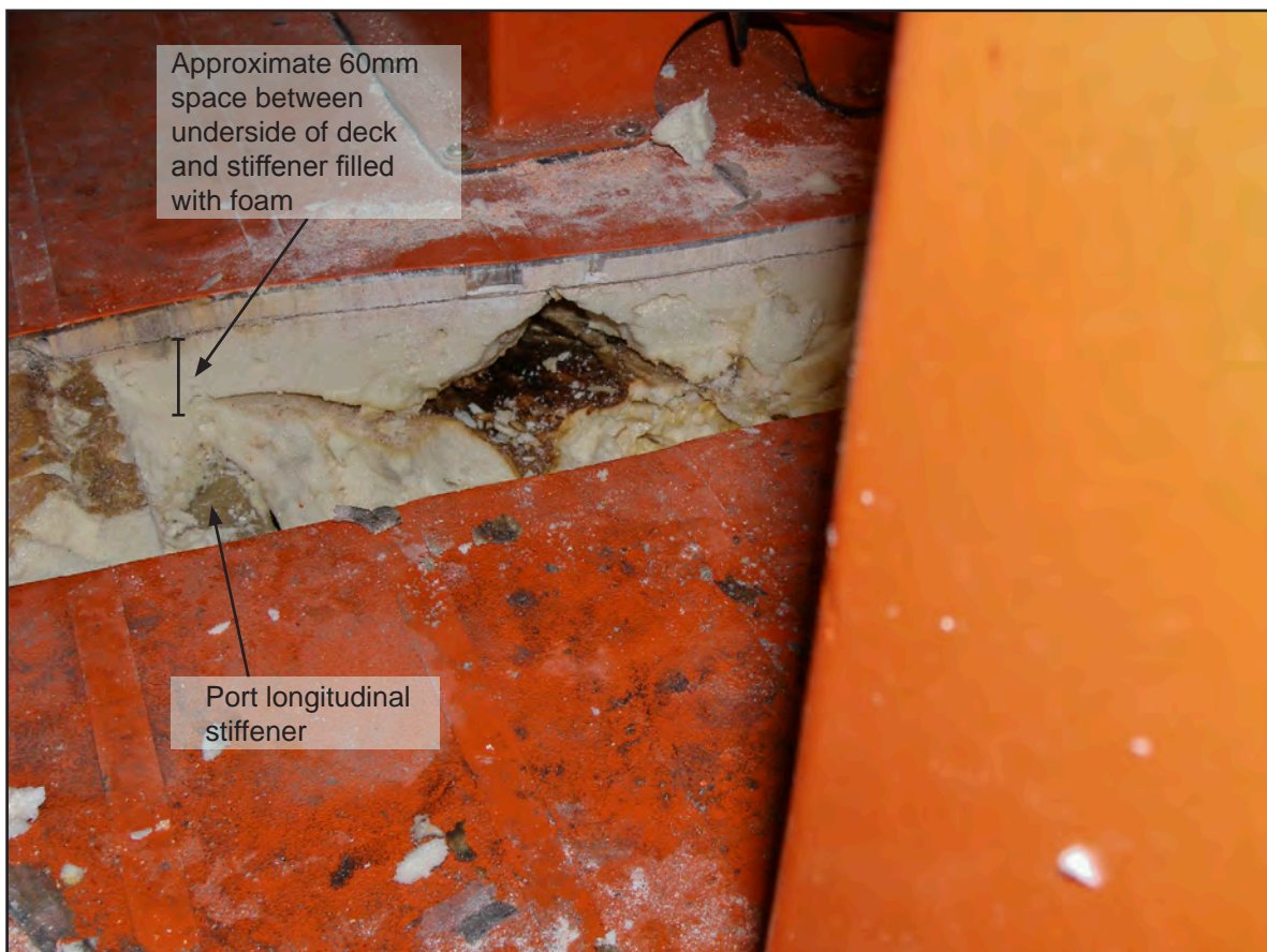
Figure 11: Degraded foam and void
