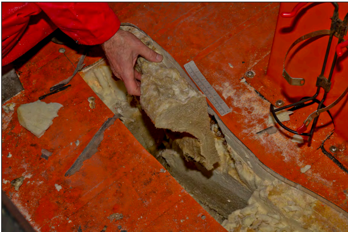
Figure 13: Void within foam
