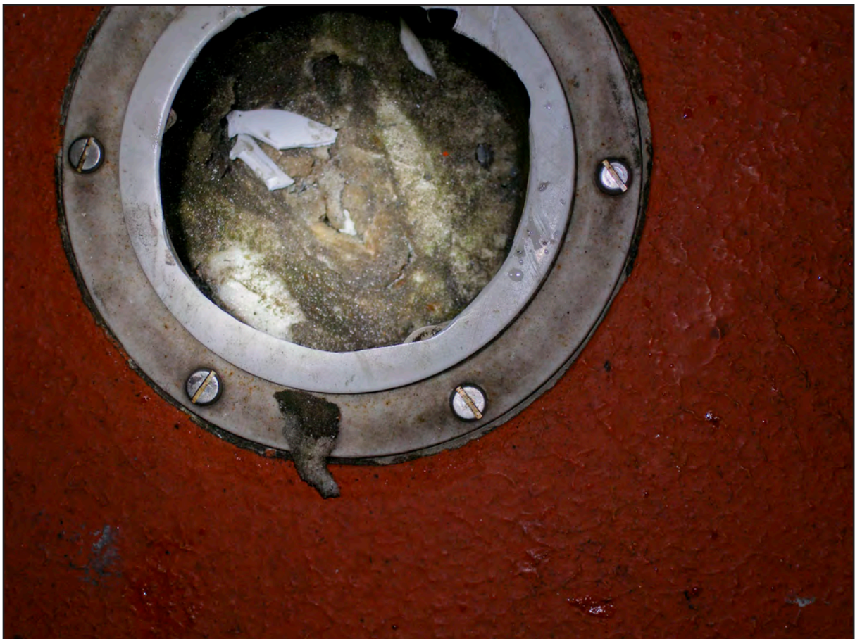
Figure 26: Inspection hatch and saturated foam
