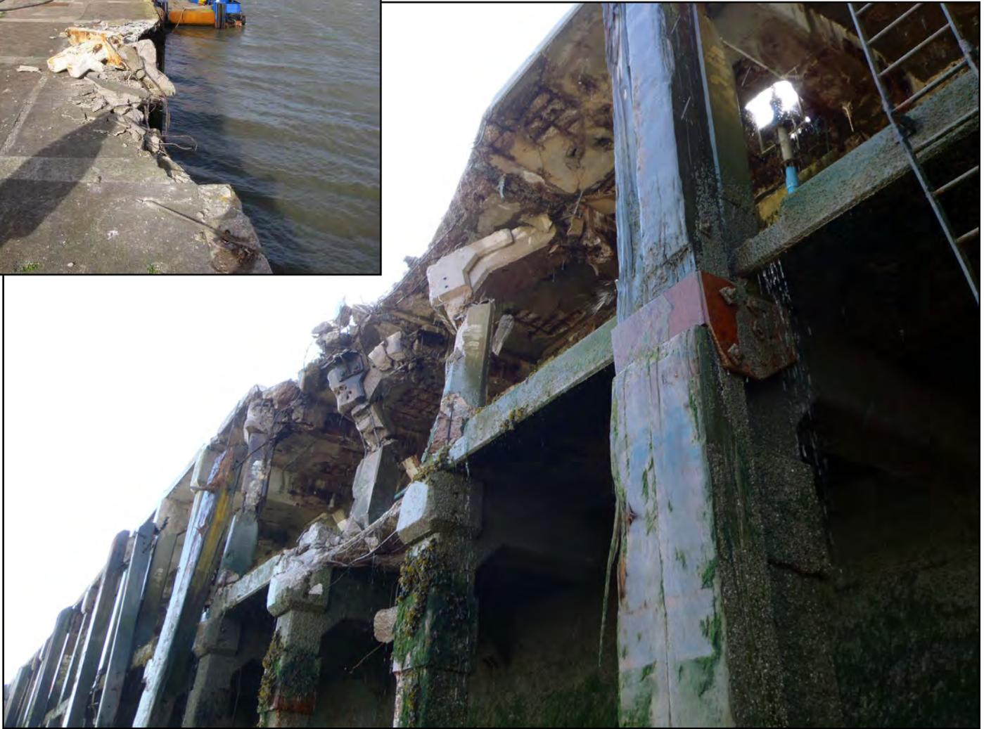
**Figure 9: Damage to South Quay**
