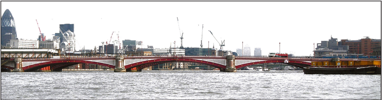
Figure 9: Blackfriars Road Bridge
