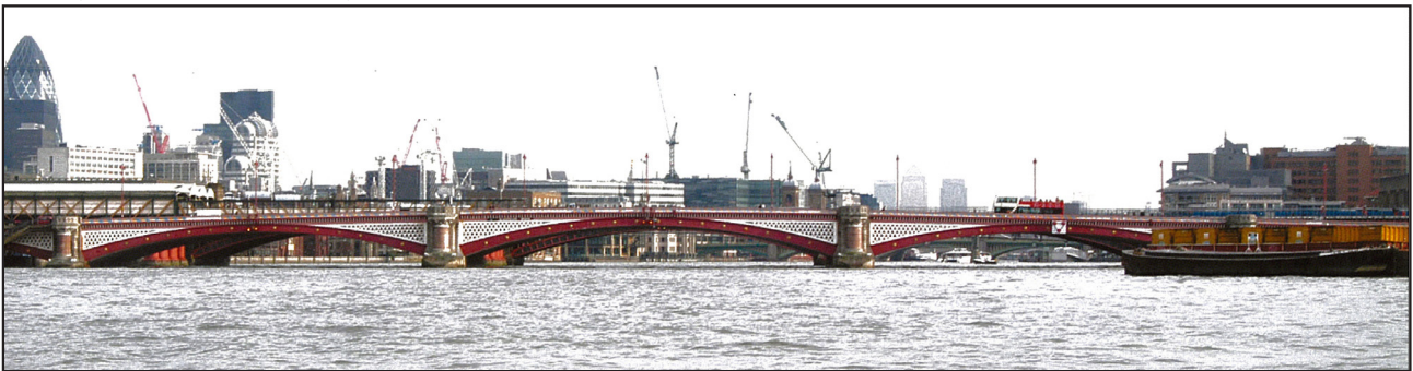
Figure 9: Blackfriars Road Bridge
