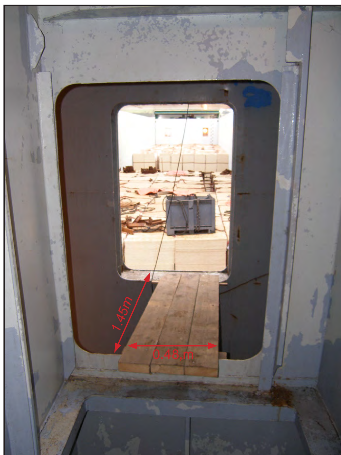
Figure 3: Wooden bridge access to hold
