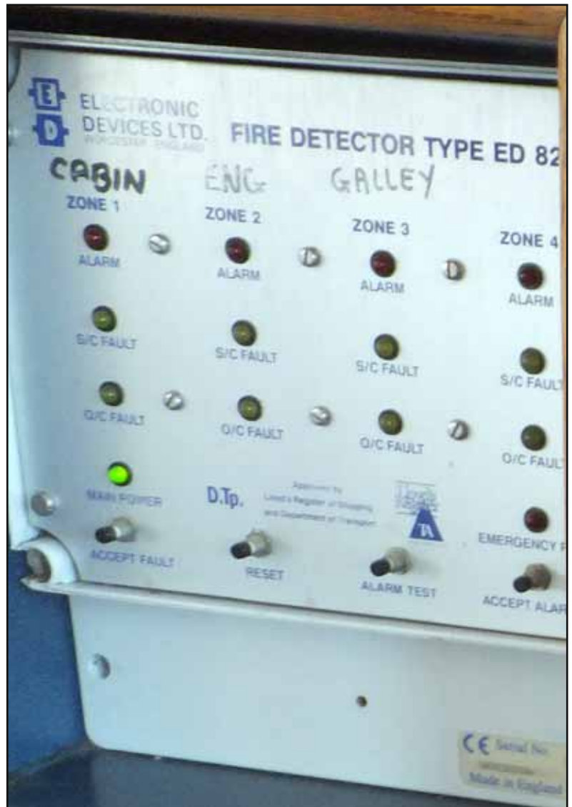
Figure 6: Fire detection system control panel ( Ocean Challenge )
