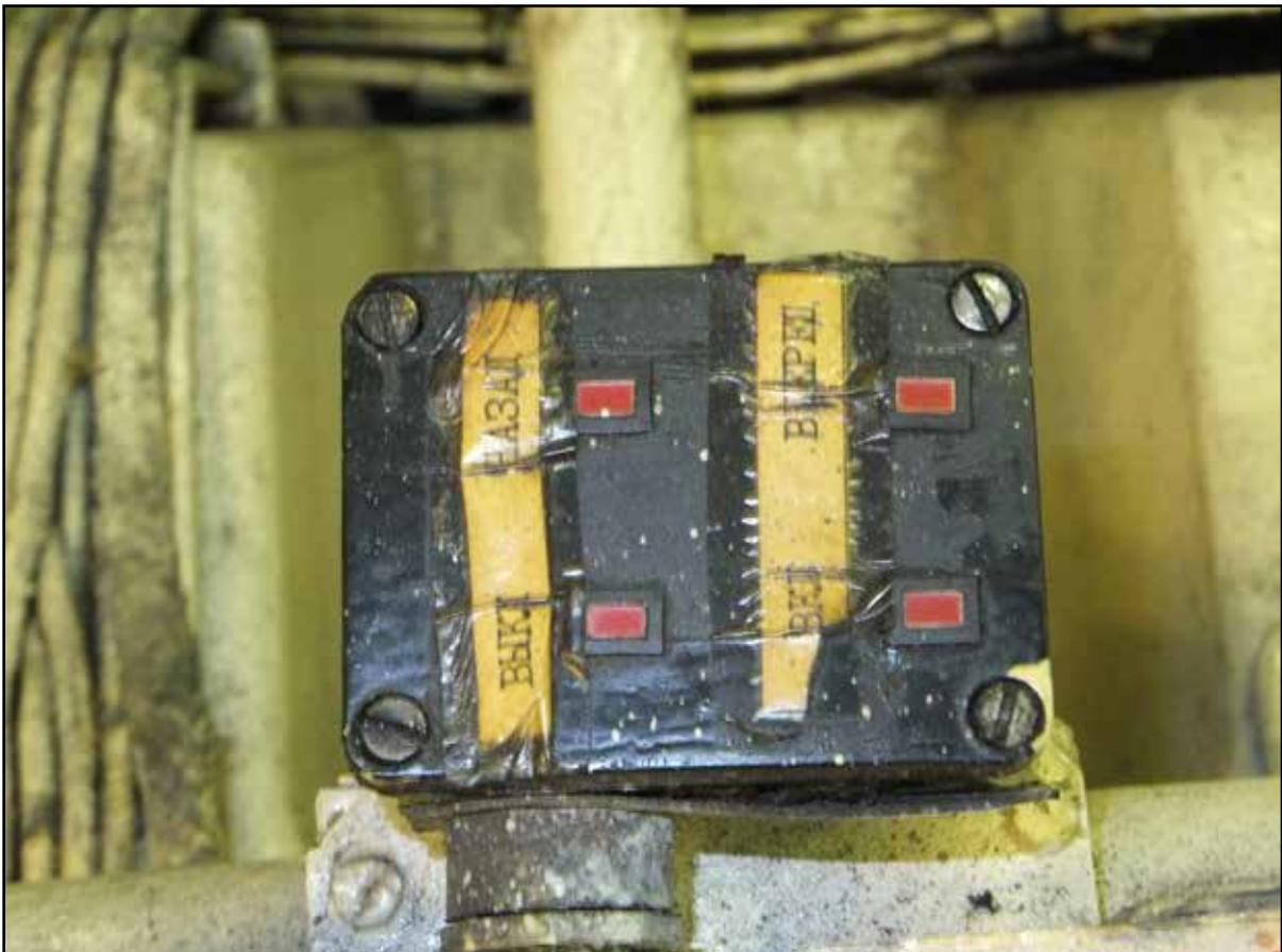
**Figure 22:** Solenoid valves indicator lamps
