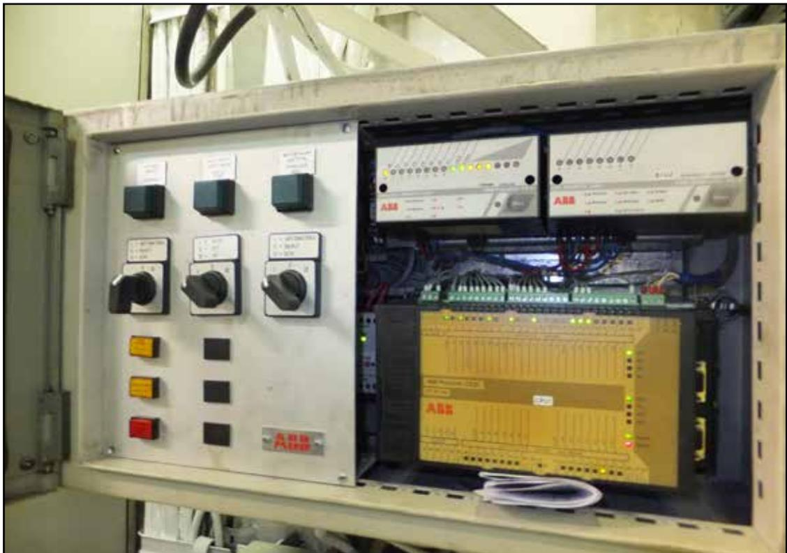
Figure 21: ABB bridge control panel
