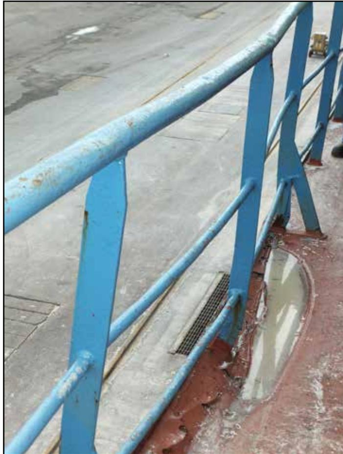
**Figure 12:** *Wilson Hawk* damage to deck starboard side
