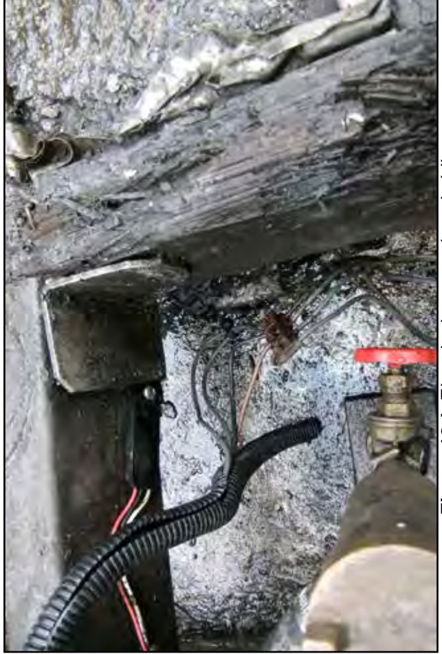
Figure 18b: Gunwhale top corrosion
