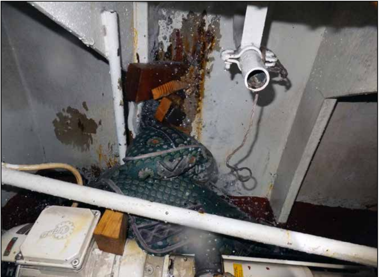
Figure 3: Damage to shell plating in engine room
