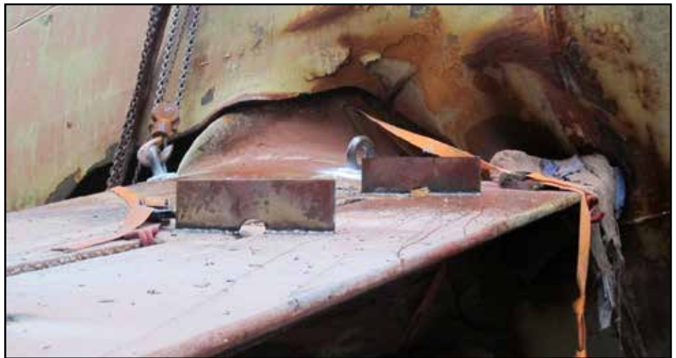
Figure 5: Port fin stabiliser and hull damage
