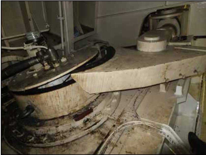
Figure 3: Port fin stabiliser head damage in separator room
