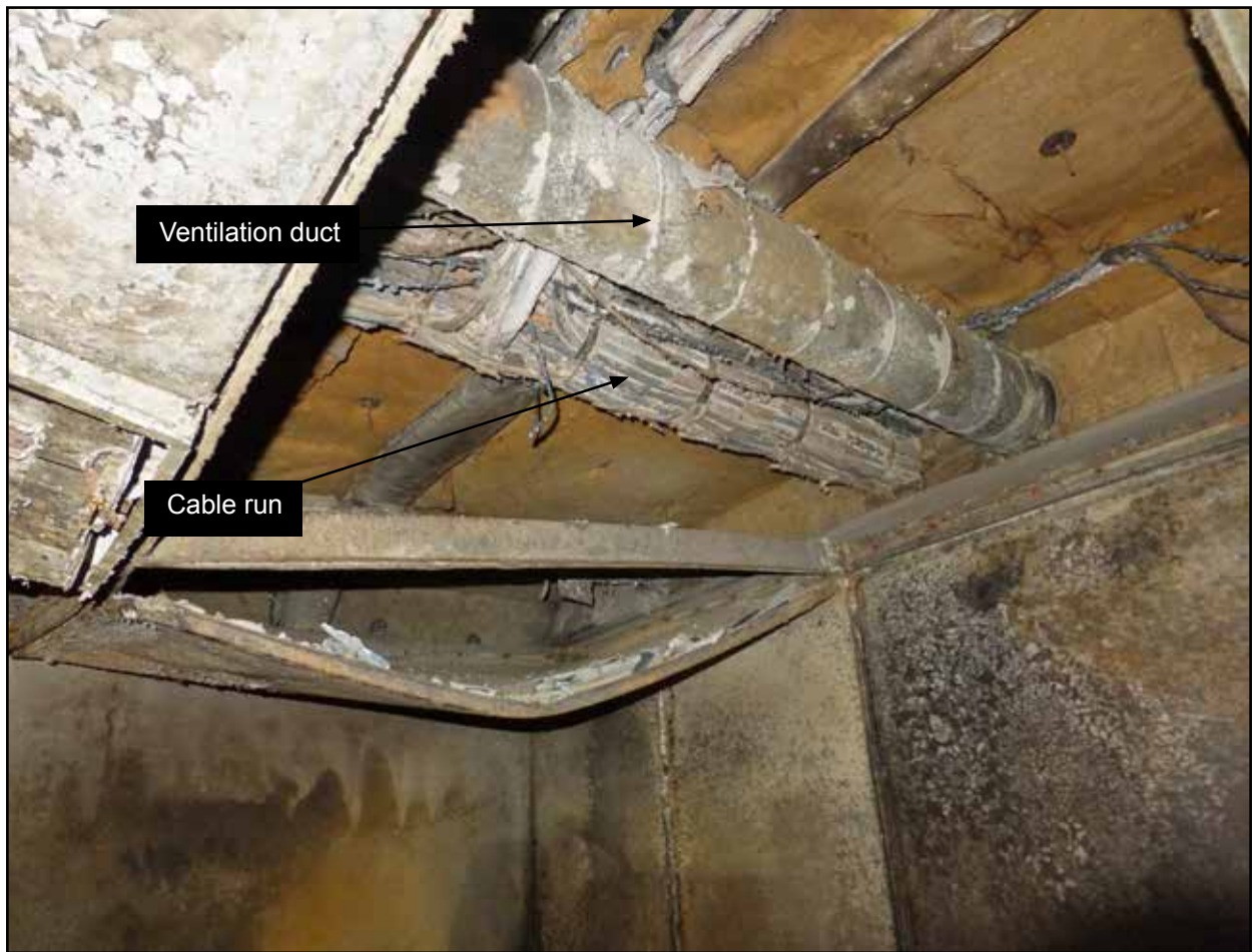
Figure 9: Void space above motorman's cabin and cable run
